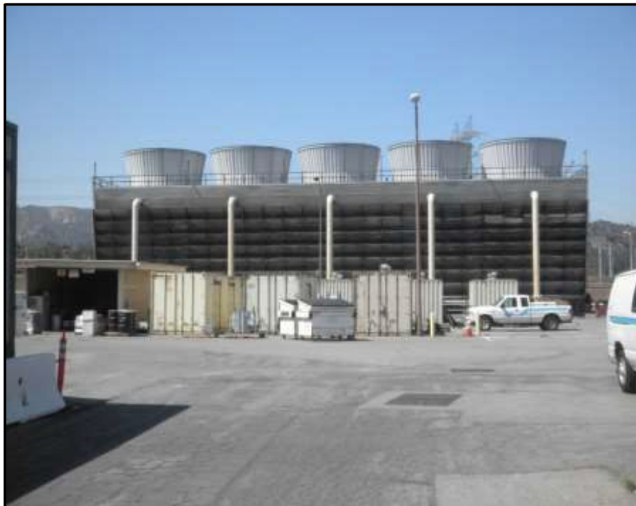
Figure 23. Cooling Tower No. 5, View Looking West (Photo by J. Terry).
