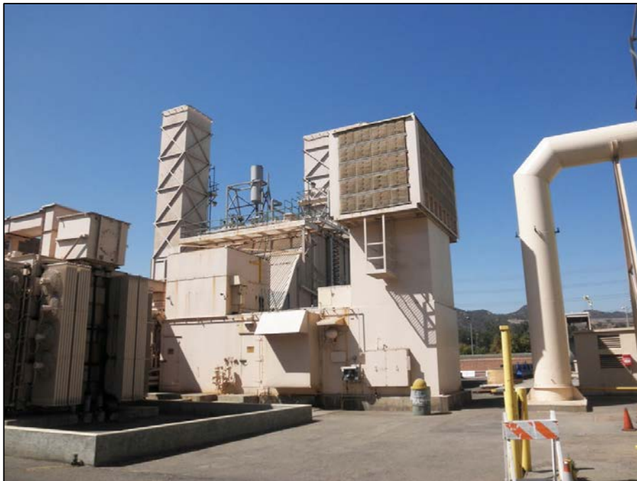
Figure 34 Unit 8A, Looking West
