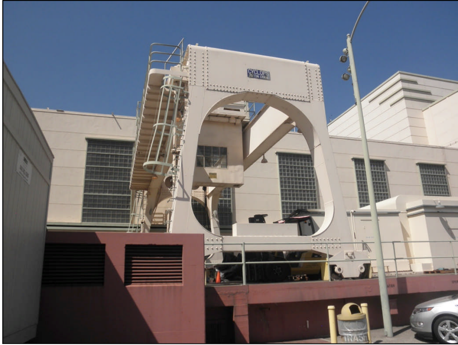
Figure 17 Grayson Boiler Building: Northeast Elevation, and Moving Crane on the Red Concrete Platform where Turbines are Located, View Looking Northwest
