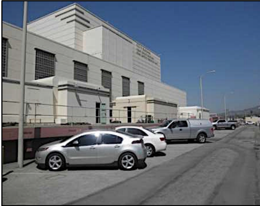
Figure 7. Grayson Boiler Building, View Looking Northwest (Photo by J. Terry).
