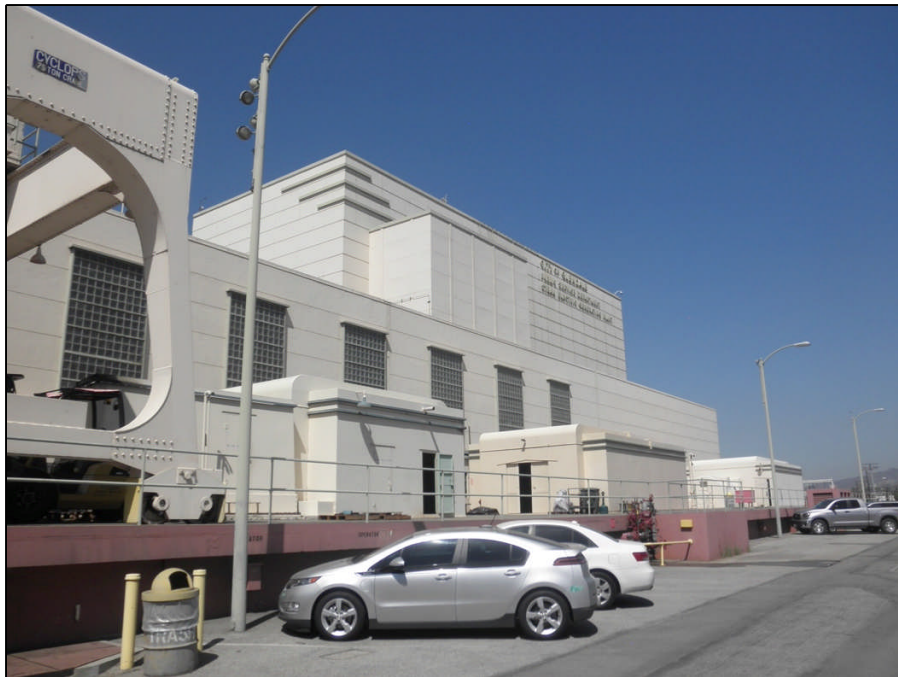
Figure 18 Grayson Boiler Building: Northeast Elevation, and its Two-Story Addition, View Looking Northwest
