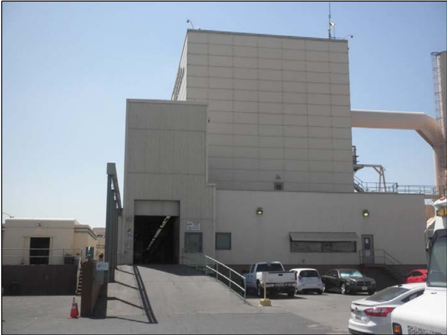
Figure 22 Grayson Boiler Building: Northwest Elevation, View Looking Southeast
