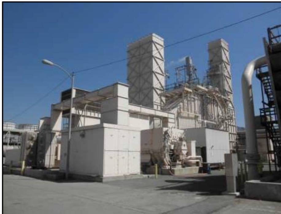
Figure 25. Units 8A & 8B, View Looking Northeast (Photo by J. Terry).
