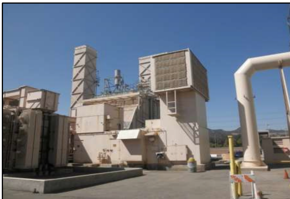
Figure 24. Unit 8A, Looking West (Photo by J. Terry).
