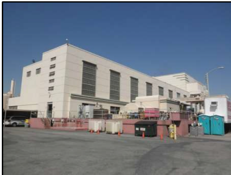
Figure 8. Grayson Boiler Building, View Looking Northwest (Photo by J. Terry).
