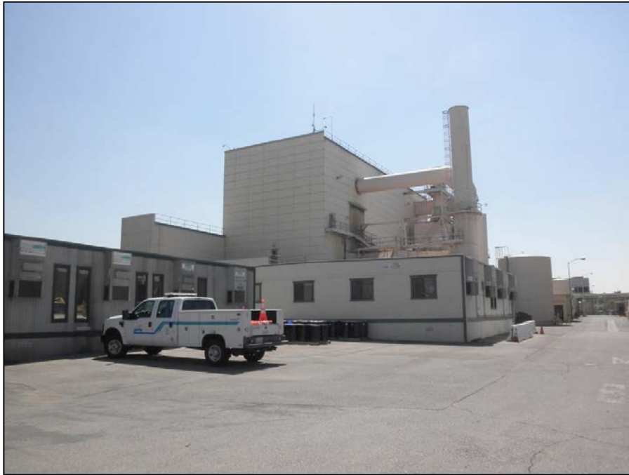
Figure 23 Grayson Boiler Building: Northwest Elevation, View Looking Southwest
