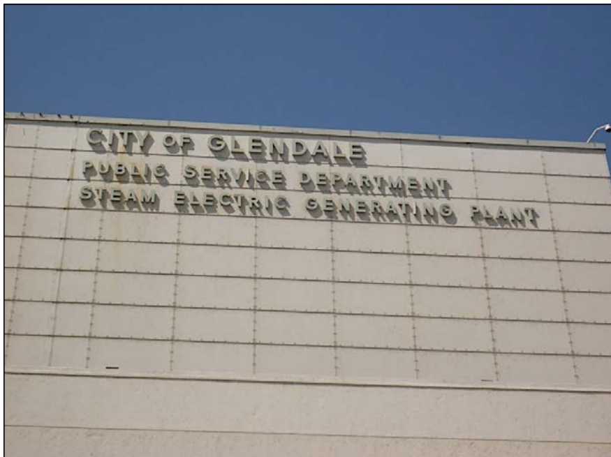
Figure 20 Grayson Boiler Building: on North End and Bronze Lettering on Asbestos Panels' States: CITY OF GLENDALE/PUBLIC SERVICE DEPARTMENT/STEAM ELECTRIC GENERATING PLANT, View Looking Northwest.
