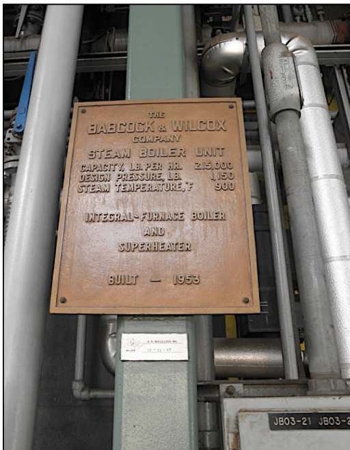
Figure 32 Grayson Boiler Building: Two Iron Mechanical Plaques. Iron Plaque for Steam Boiler Unit, Records Babcock Wilcox of New York in 1953 near Boiler 1A (left); Two Iron Plaques on Boiler 1A Record Steam Generator of New York from Combustion Engineering Company, Inc., built in 1940
