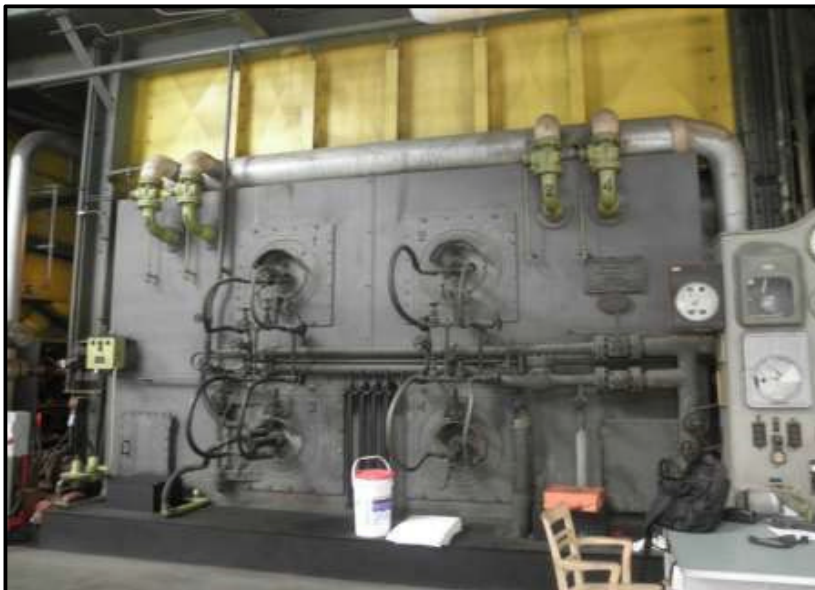
Figure 17. View of Boiler 1B, Looking West (Photo by J. Terry).
