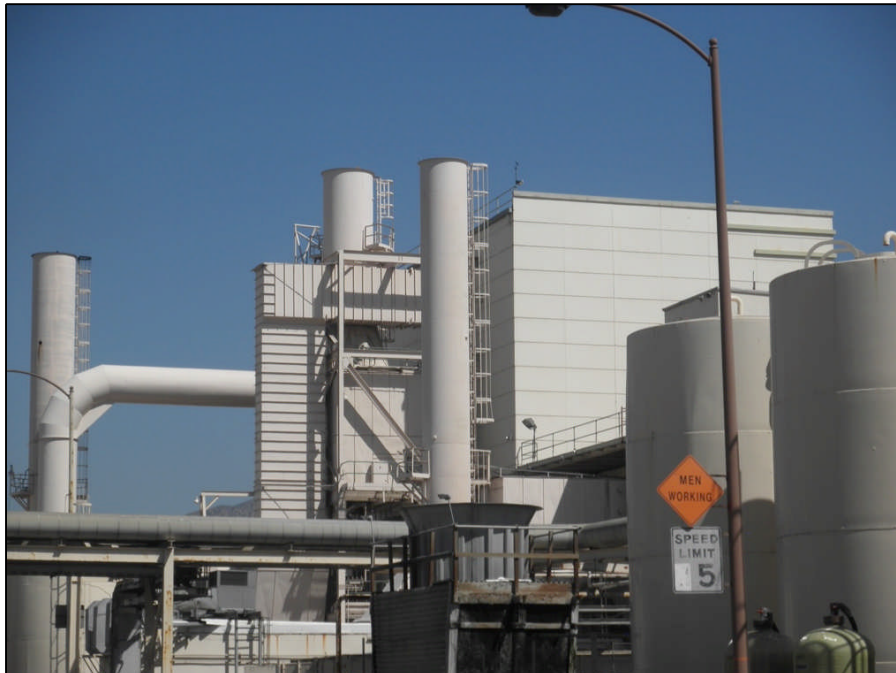
Figure 24 Grayson Boiler Building: Northwest Elevation, and Additions on the Two-Story Component, View Looking Southwest
