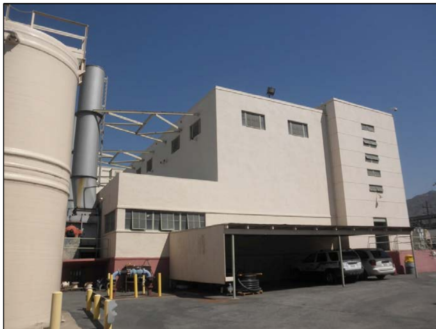
Figure 26 Grayson Boiler Building: Southeast Elevation, View Looking Northeast
