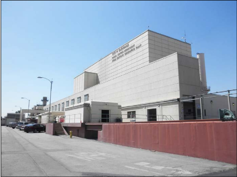
Figure 21 Grayson Boiler Building: Northwest Elevation, View Looking Southeast
