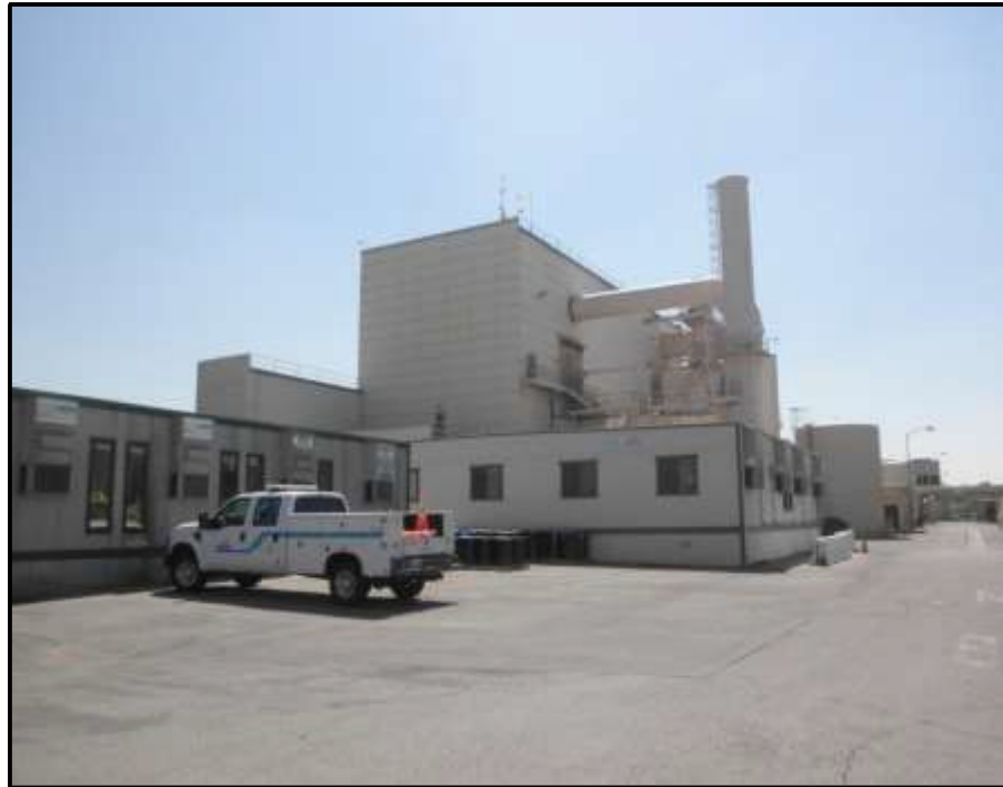
Figure 9. Grayson Boiler Building, View Looking Southwest (Photo by J. Terry).
