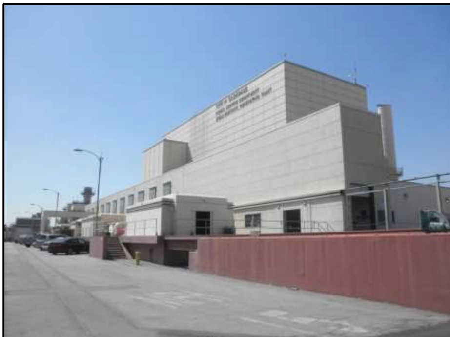
Figure 10. Grayson Boiler Building, View Looking Southeast (Photo by J. Terry).
