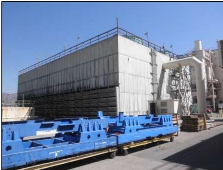
Figure 22. Cooling Tower No. 4, View Looking Northeast (Photo by J. Terry).
