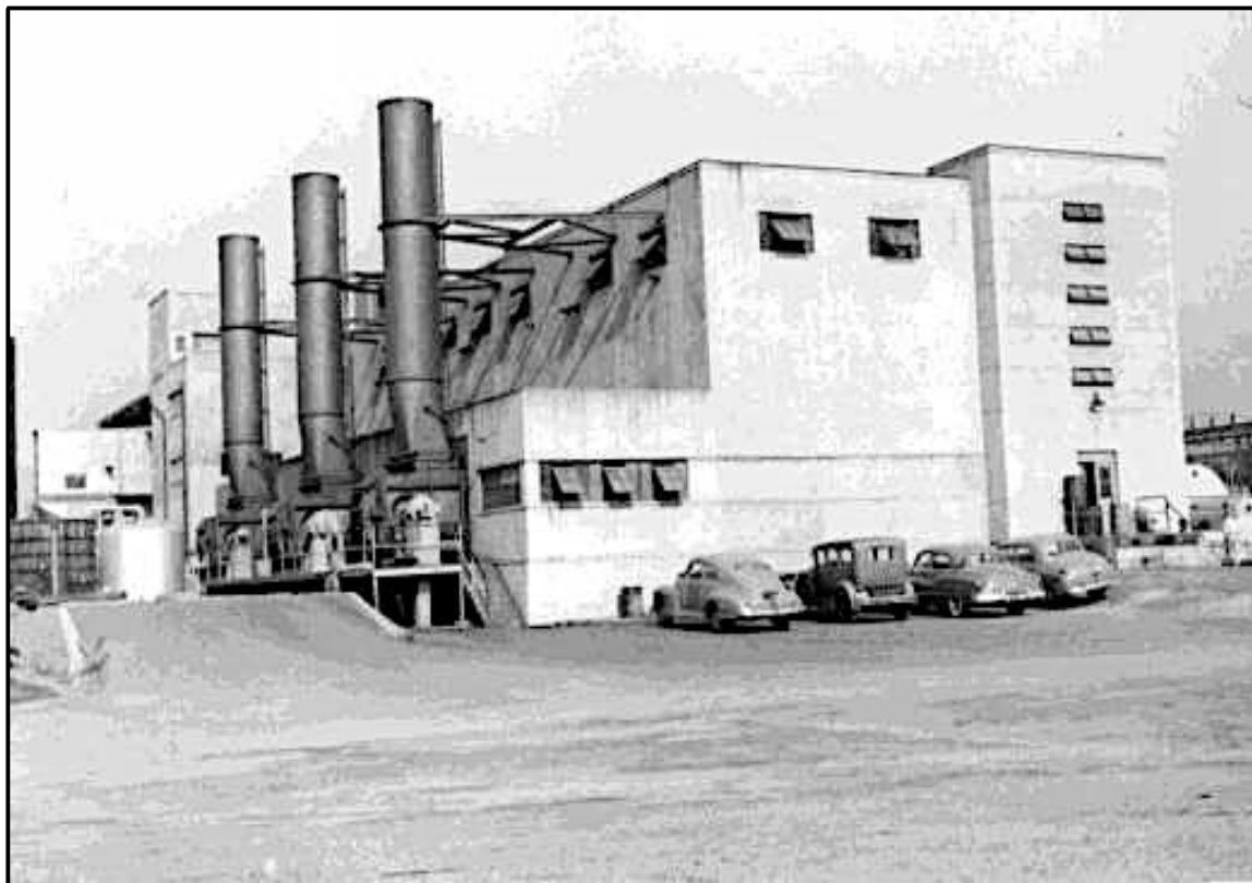
Figure 6. Grayson Power Plant c. 1950 (Collection of the City of Glendale Water and Power).
