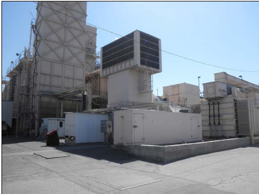
Figure 36 Units 8A, 8B, & 8C, View Looking Southeast
