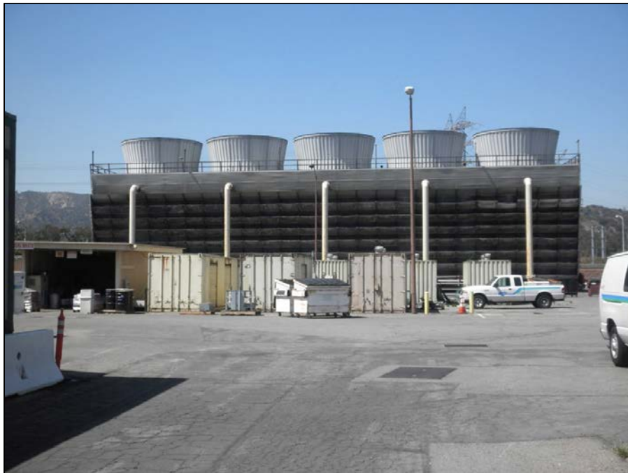
Figure 41 Cooling Tower No. 5, View Looking West
