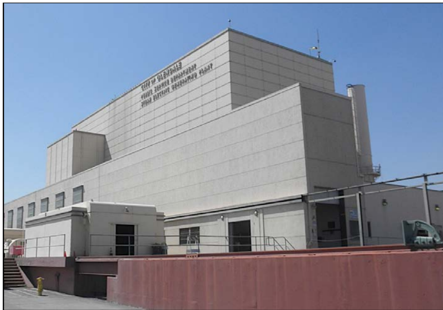
P5a. Photograph or Drawing (Photograph required for buildings, structures, and objects.)
