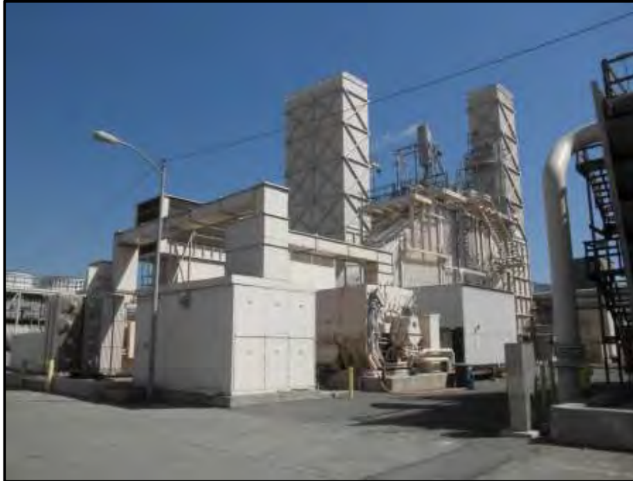
Photograph 10. Units 8A & 8B, View Looking Northeast (Photo by J. Terry).
