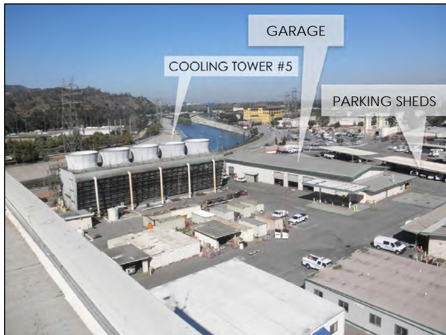
Figure 4 Overview of Project Area from Roof of Grayson Boiler Building Looking Northwest
