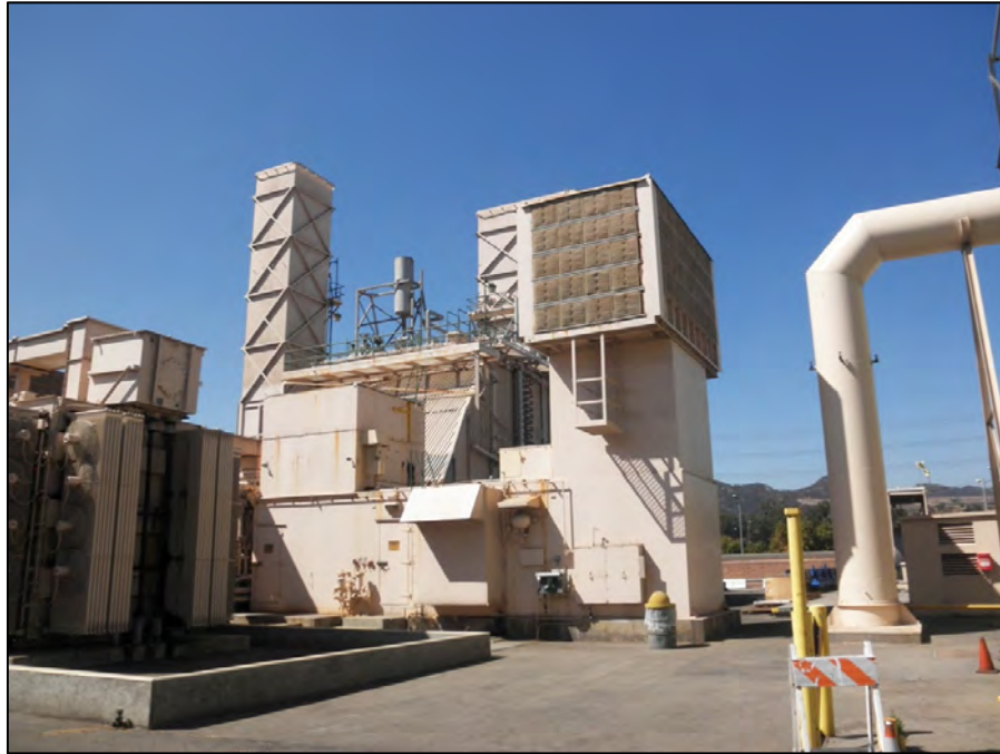
Figure 34 Unit 8A, Looking West
