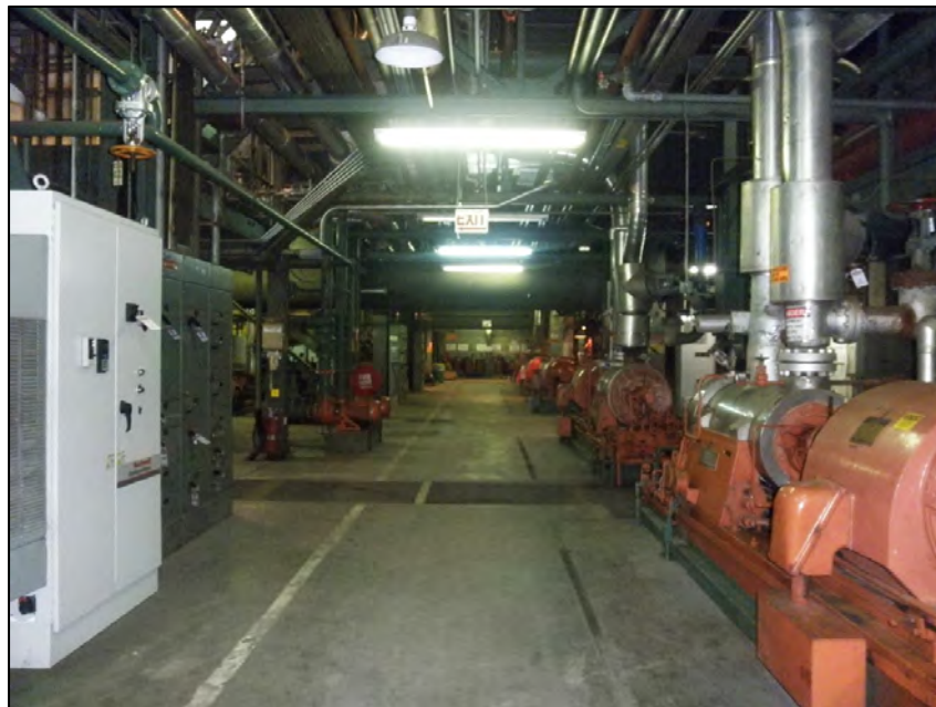
Figure 27 Grayson Boiler Building: Interior Overview of Basement Floor Level, View Looking North
