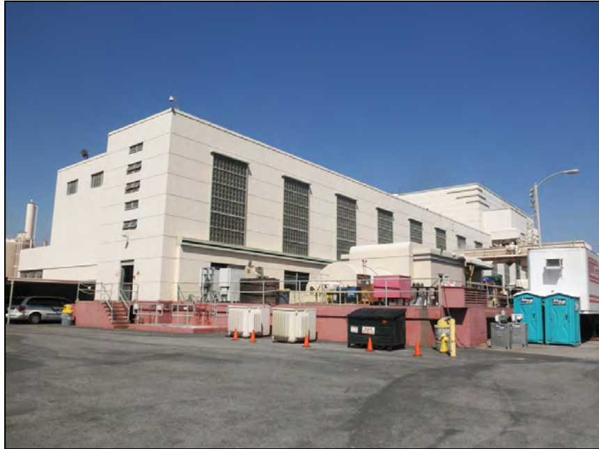
Figure 16 Grayson Boiler Building: Northeast Elevation, View Looking Northwest
