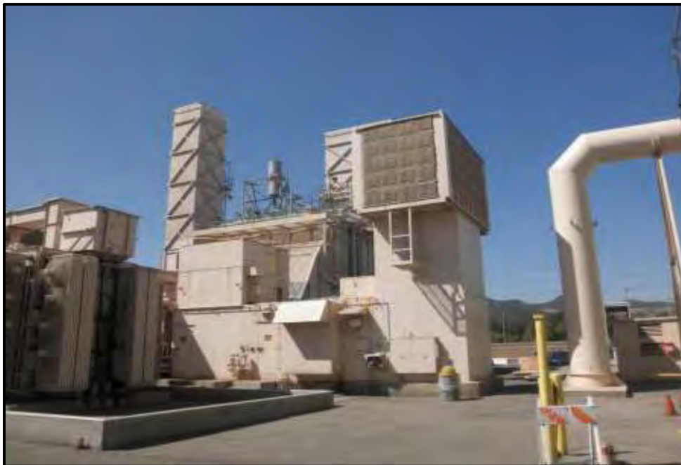
Photograph 9. Unit 8A, Looking West (Photo by J. Terry).
