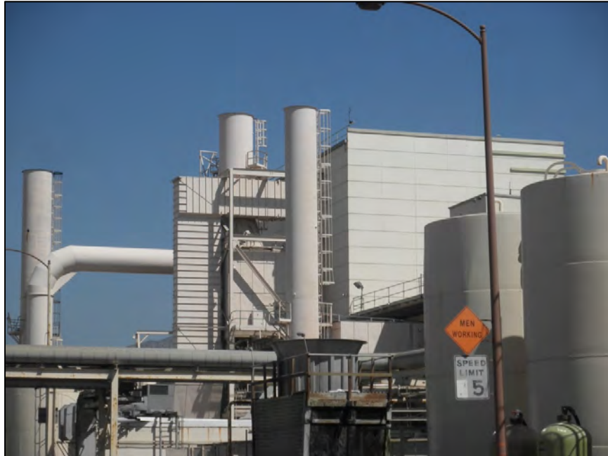
Figure 24 Grayson Boiler Building: Northwest Elevation, and Additions on the Two-Story Component, View Looking Southwest
