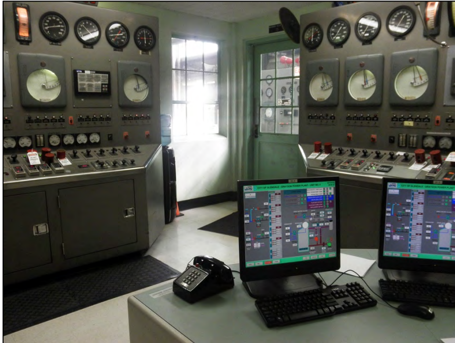
Figure 30 Grayson Boiler Building: Interior of Control Room, View Looking Northwest
