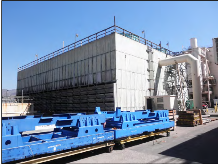
Figure 40 Cooling Tower No. 4, View Looking Northeast
