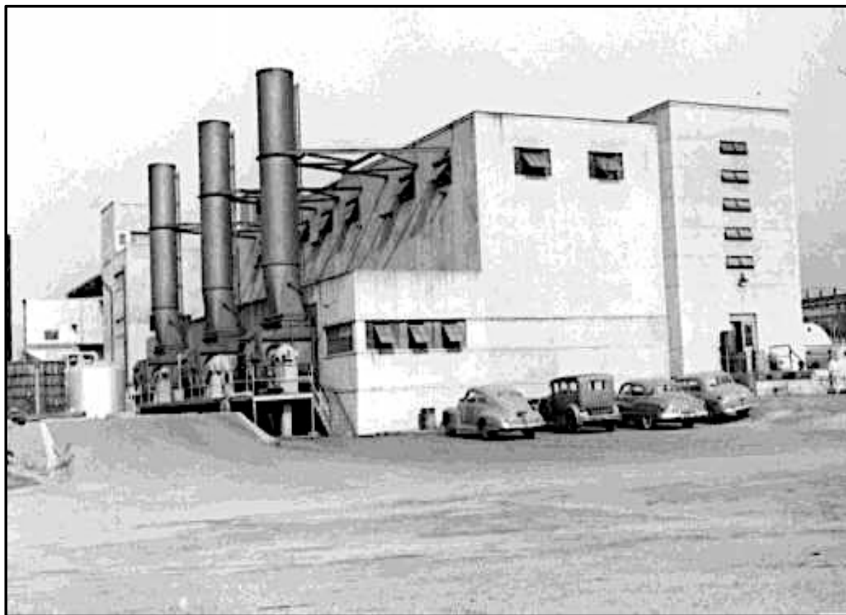
Figure 14 Grayson Power Plant c. 1950 (Collection of the City of Glendale Water and Power)
