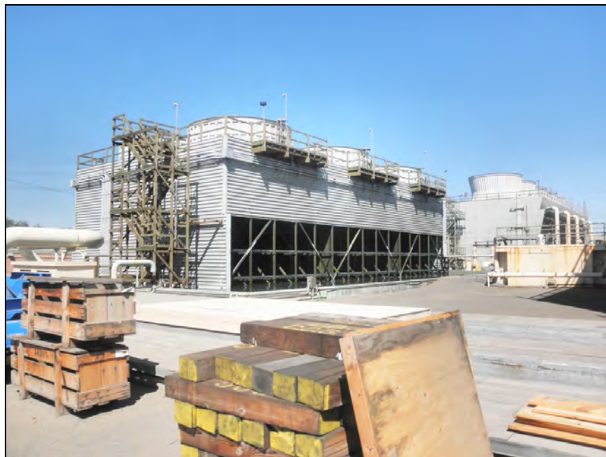
Figure 39 Cooling Tower No. 3 (Cooling Tower No. 5 in Background), View Looking Northwest
