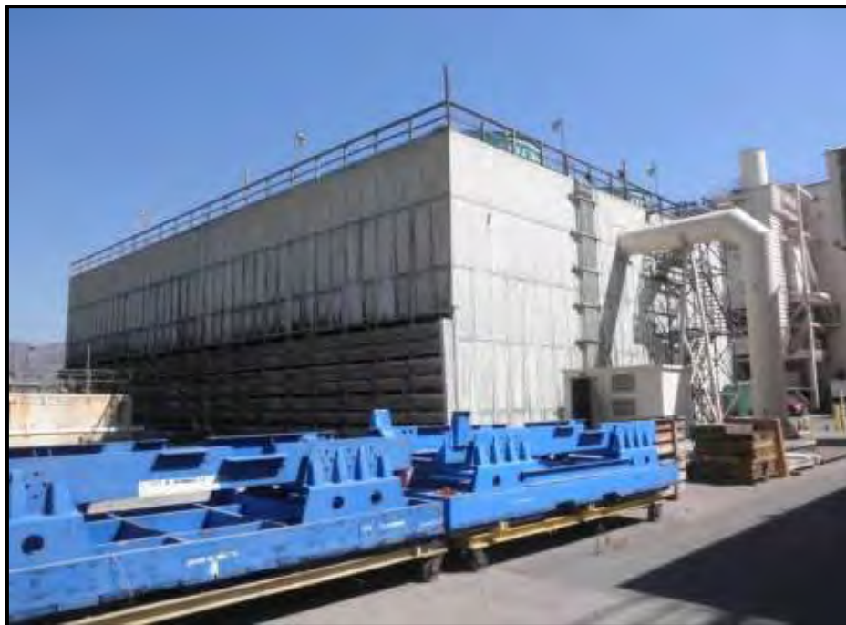
Photograph 14. Cooling Tower No. 4, View Looking Northeast (Photo by J. Terry).
