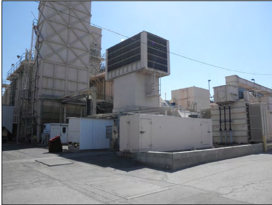
Figure 36 Units 8A, 8B, & 8C, View Looking Southeast
