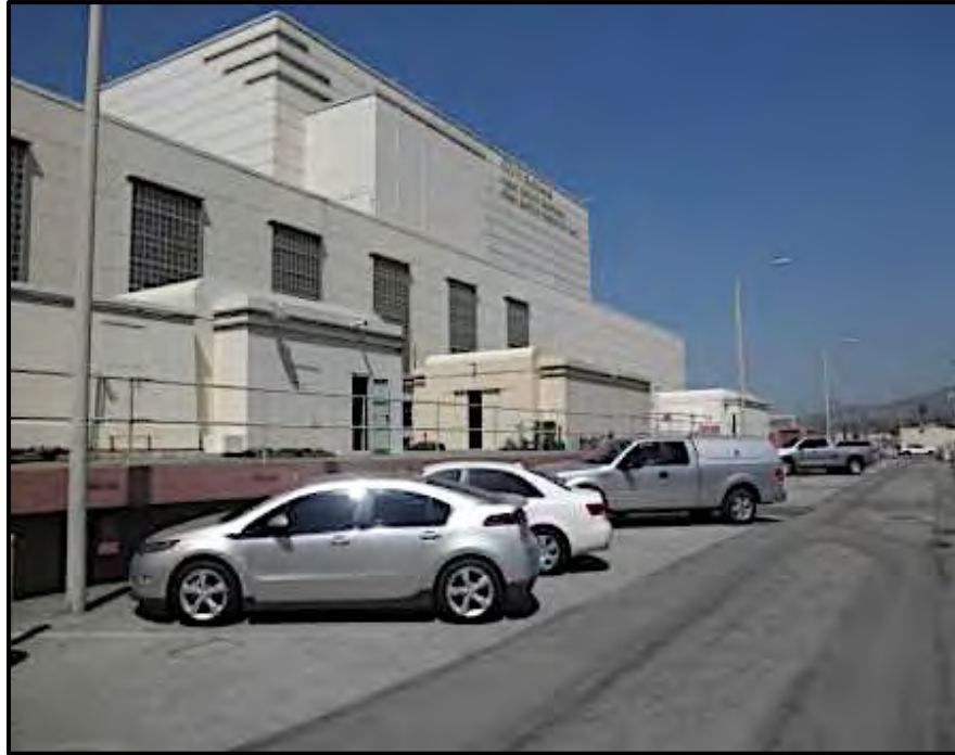
Photograph 2. Grayson Boiler Building, View Looking Northwest (Photo by J. Terry).
