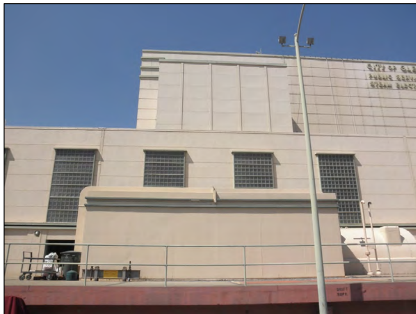
Figure 19 Grayson Boiler Building: Looking at Original Glass Block Windows and a Turbine at North End of Northeast Elevation, View Looking Northwest
