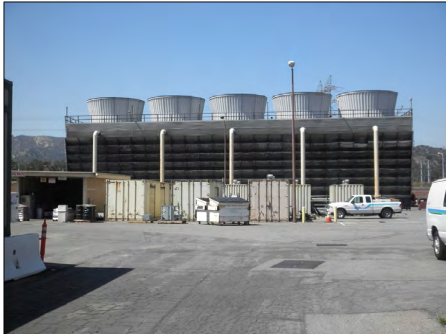
Figure 41 Cooling Tower No. 5, View Looking West
