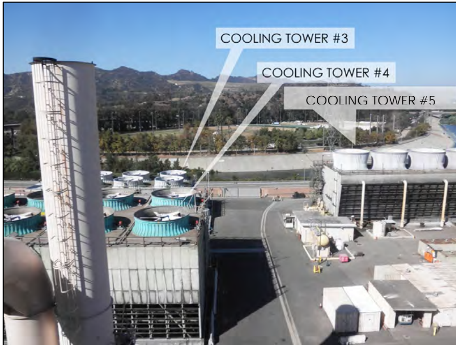
Figure 5 Overview of Project Area from Roof of Grayson Boiler Building Looking West
