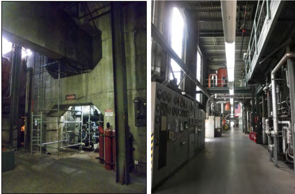
Figure 28 Grayson Boiler Building: Basement Level Depicting Concrete Structure Below Turbine and Generator 1, View Looking Northeast (left); Overview of Main Level, View Looking South (right)
