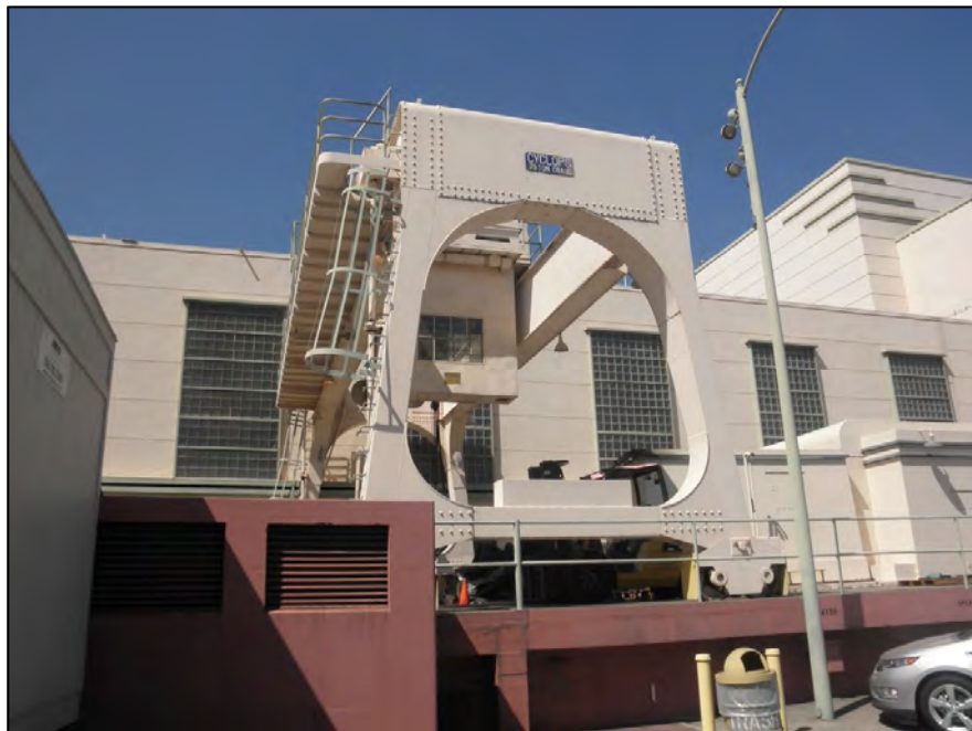
Figure 17 Grayson Boiler Building: Northeast Elevation, and Moving Crane on the Red Concrete Platform where Turbines are Located, View Looking Northwest
