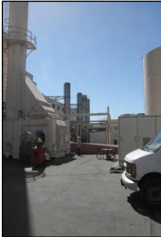
Photograph 6. Boiler Stacks (Boilers 1 and 2 Center Rear of Photograph; Boiler 3 to Left), View Looking South. (Photo by J. Terry).
