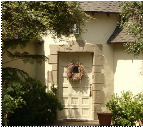
Above: This entrance exhibits detail through its symmetrical patterning of stone quoining and paneled door.
