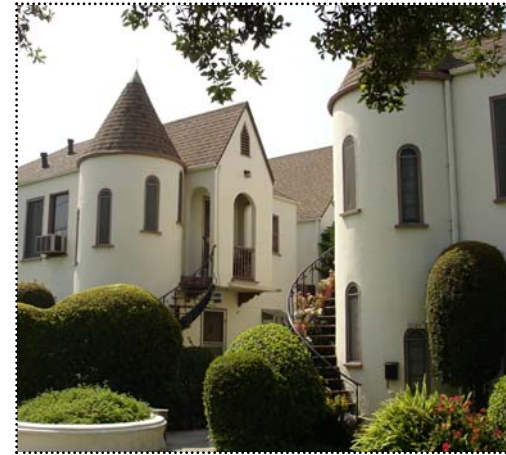
Above: The multi-family apartments give the appearance of being large single-family homes. The landscaping and multiple stair entries lend to the character of the complex.
