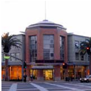
TOP LEFT: Entry corner indicated by architectural tower and primary entrance
