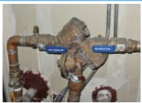
Approved backflow prevention devices installed at water main connections to a high-rise building.
