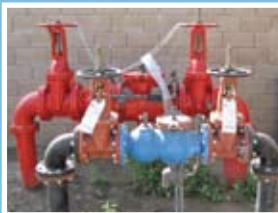
Approved backflow prevention devices installed at water main connections to a high-rise building.
