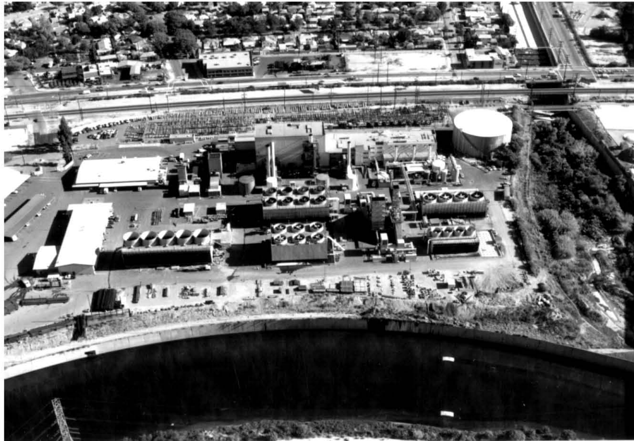
GRAYSON POWER PLANT
