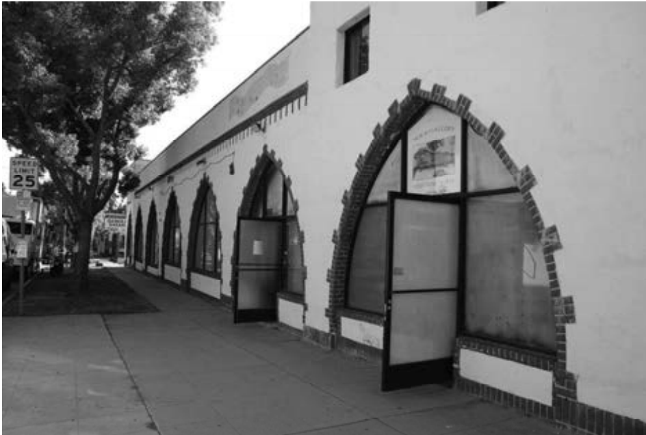
Partial South Façade, South Central Avenue, looking west. Historic Resources Group, August 2013.
