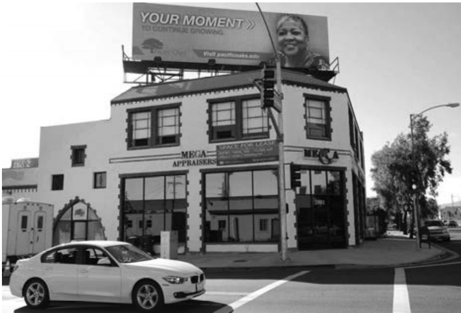
Partial South Façade, South Central Avenue, looking north. Historic Resources Group, August 2013.
