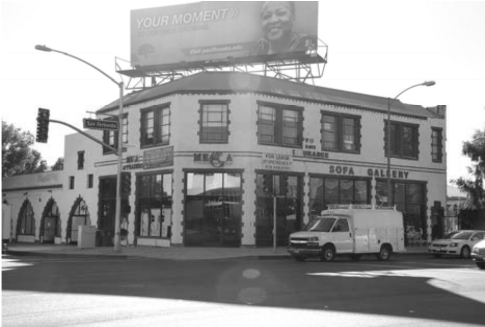
East Façade and partial South Façade, San Fernando Road and South Central Avenue, looking northwest. Historic Resources Group, August 2013.
