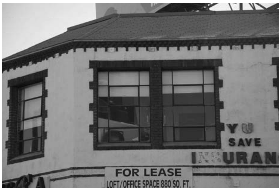
Detail of windows, East Façade. Historic Resources Group, August 2013.
