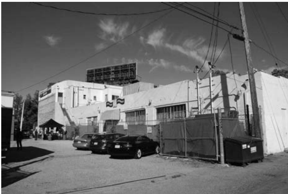
North Façade, looking southeast. Historic Resources Group, August 2013.
