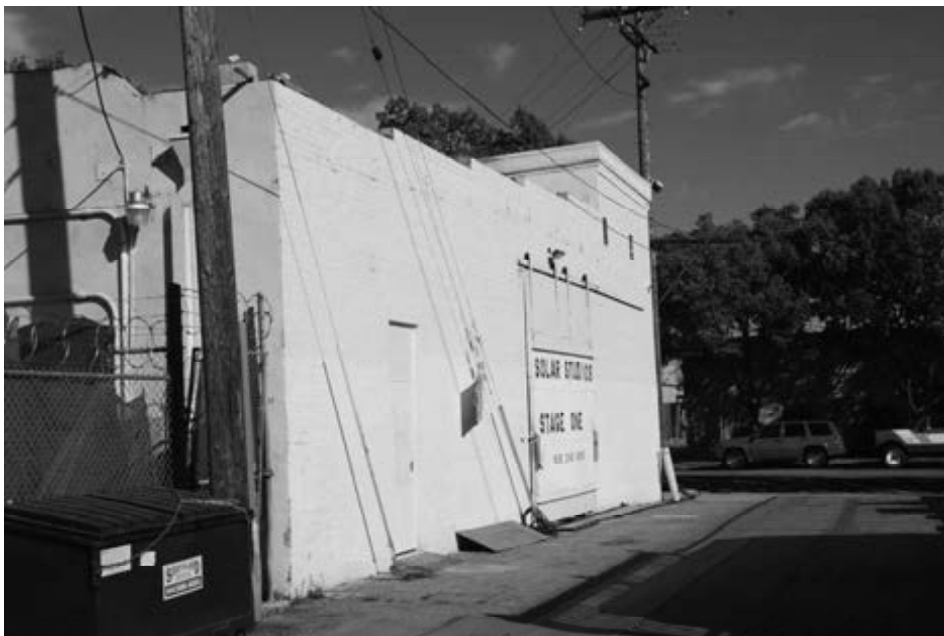
West Façade, alley, looking southeast. Historic Resources Group, August 2013.
