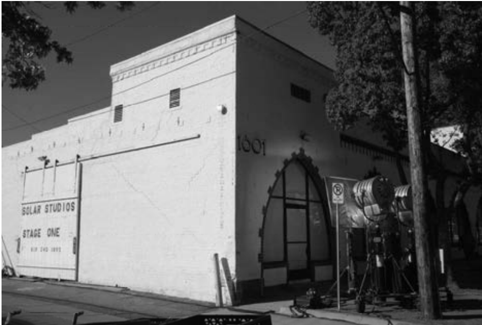
Southwest corner, South Central Avenue, looking northeast. Historic Resources Group, August 2013.
