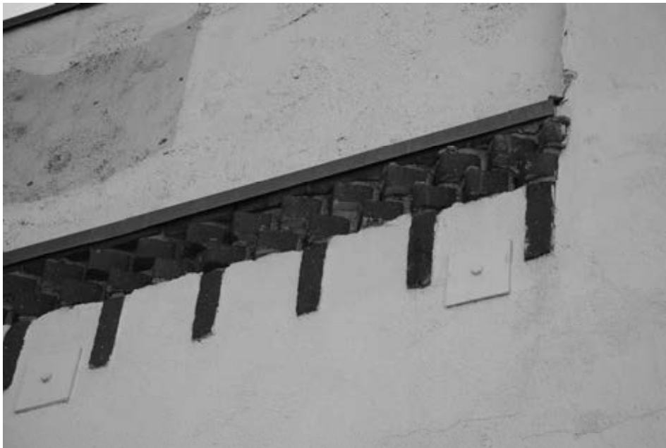
Detail of brick eave cornice, South Façade. Historic Resources Group, August 2013.
