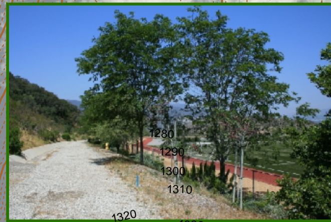
Looking West along the existing service road
