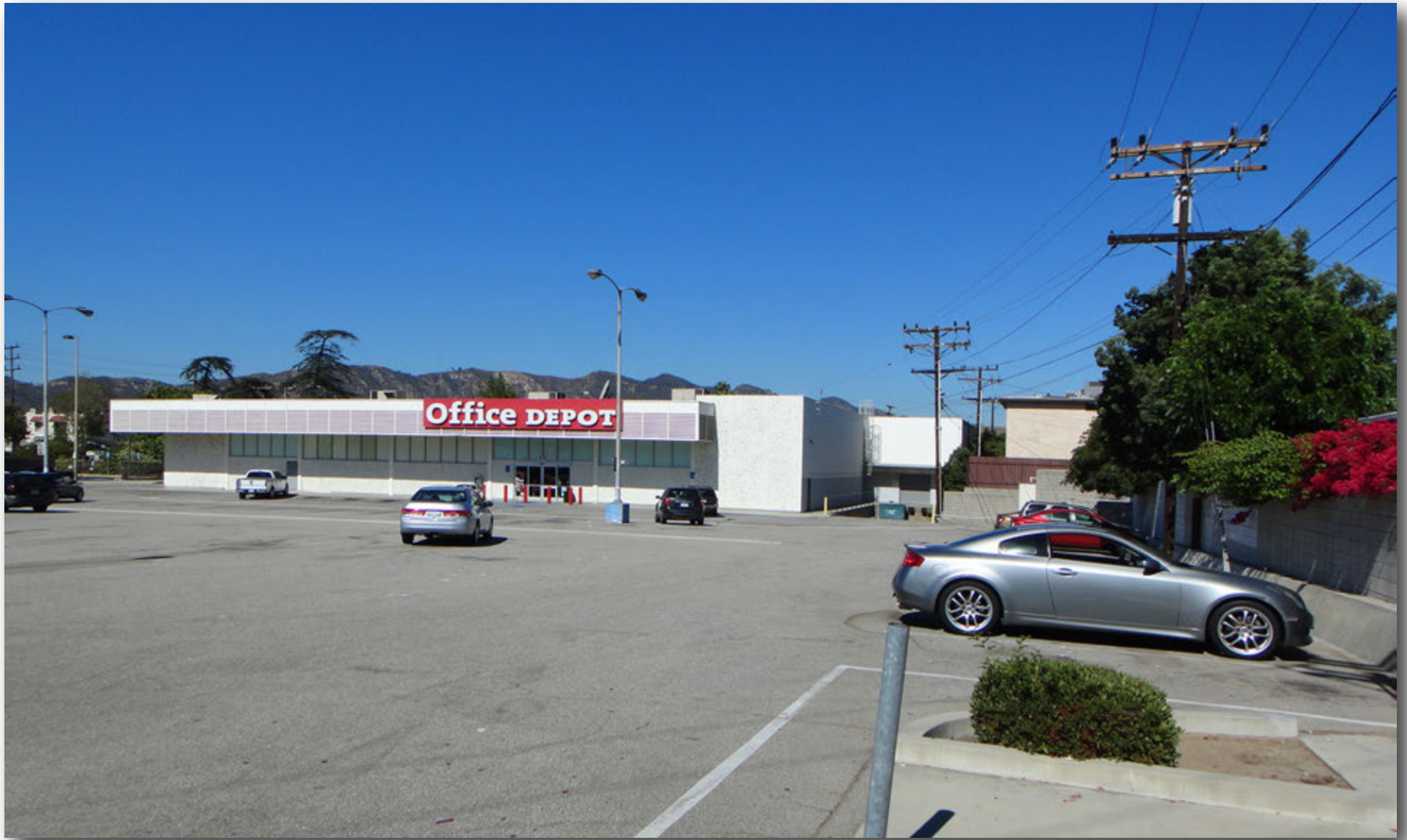
Located on northeast corner of the Project site looking west from Pacific Avenue
