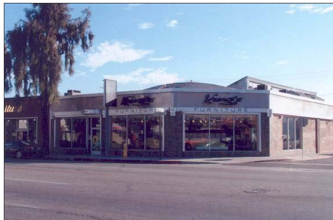
After façade grant improvement
