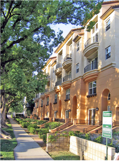
ABOVE: The Madison Avenue development in Pasadena.
