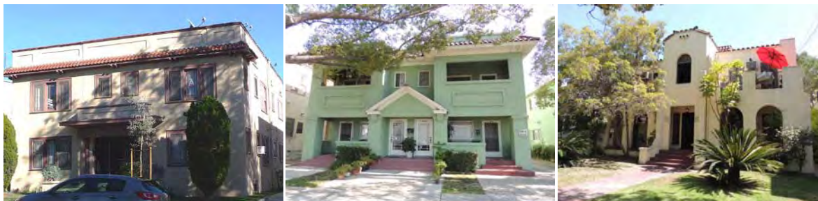
1920s apartment houses in South Glendale, L to R: 618 S. Louise, 106-108 Lomita Avenue, 110 California Avenue. Photographs 2014; Historic Resources Group.
