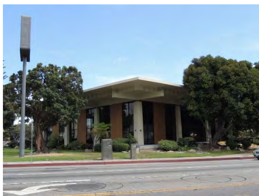
Prudential Savings and Loan (now Chase Bank) 500 N. Glendale Boulevard. Photograph 2014, Historic Resources Group.
