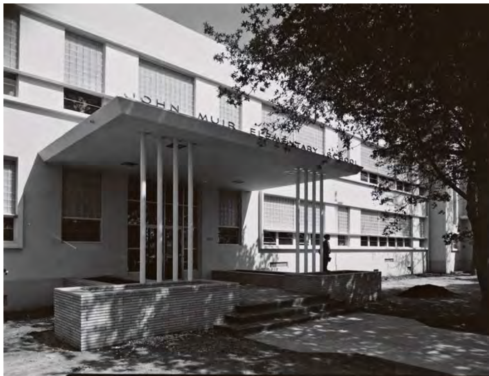
John Muir Elementary School (c. 1951, Orr, Strange and Inslee) at 1017 S. Glendale Avenue. Photo: Julius Shulman. Source: The J. Paul Getty Trust, The Getty Research Institute.
