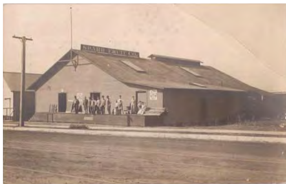
The Sparr Fruit Packing Company (demolished). Source: Michael Morgan.
