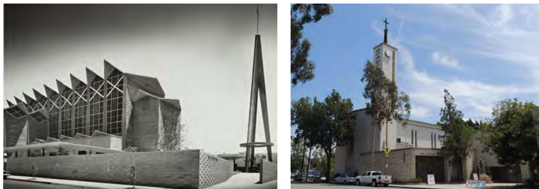
L: First United Methodist Church (1961, Flewelling and Moody). Photo: Julius Shulman. Source: The J. Paul Getty Trust, The Getty Research Institute. R: First Lutheran Church (1326 Colorado). Photograph 2014; Historic Resources Group.
