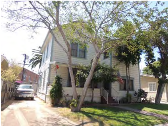
227 Everett St. Source: Historic Resources Group, July 2014.
