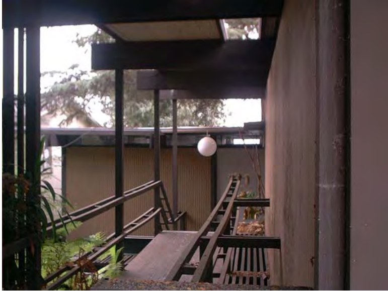
Holmes House, Raul Garduno, 1964, 1515 Corona. Photograph 2008; The Glendale Historical Society.
