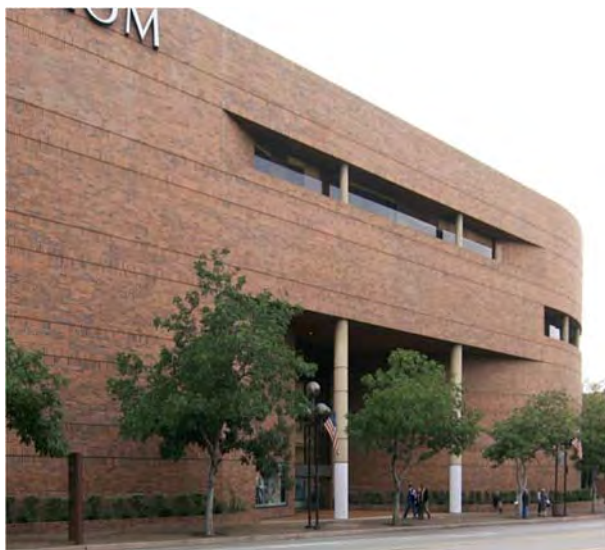
Glendale Galleria Phase II (1981, Symonds/Feola/Deenihan Architects) matched the red brick facades of Galleria Phase I.
