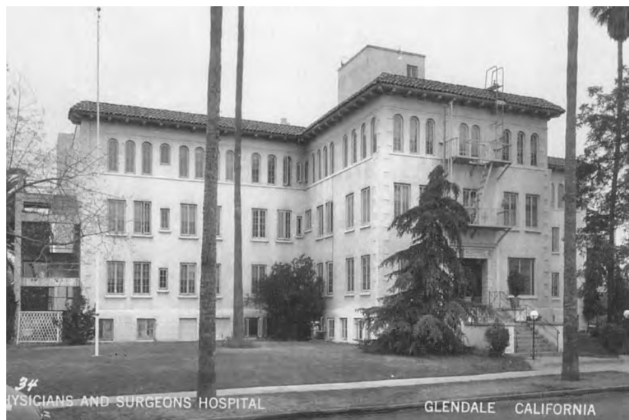
Physicians and Surgeons Hospital (1926, Roth and Parker; demolished) on the north side of W. Laurel Street. The four-story Mediterranean Revival-style building cost $250,000. Source: Special Collections Room, Glendale Public Library.
