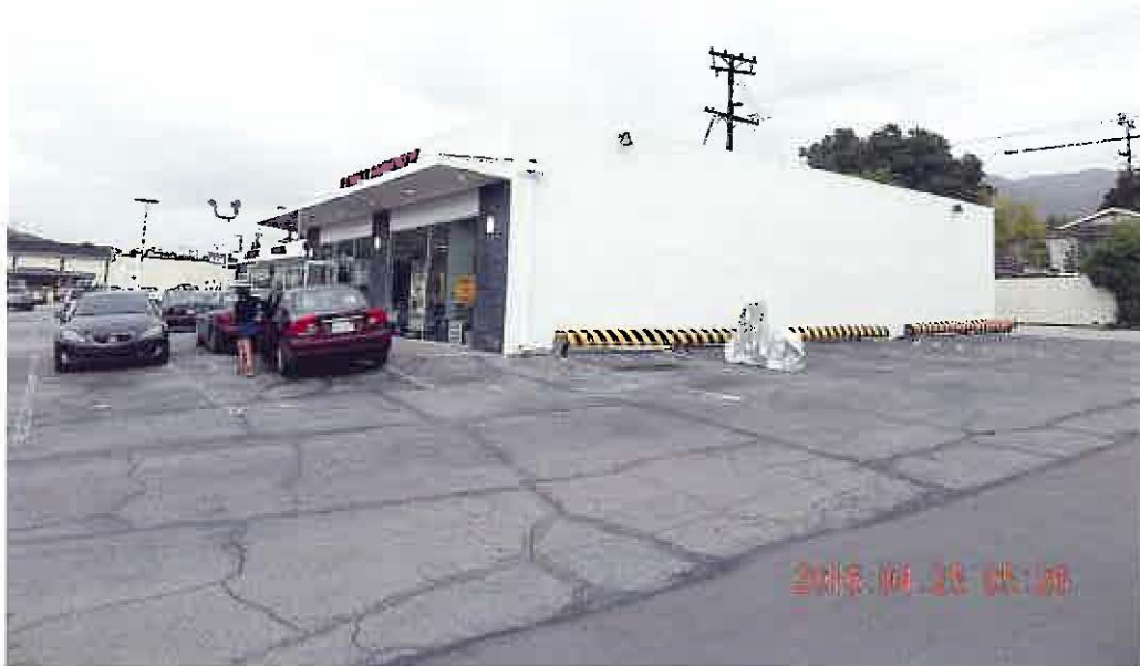
BLDG. SOUTH-EAST CORNER, from side parking.
