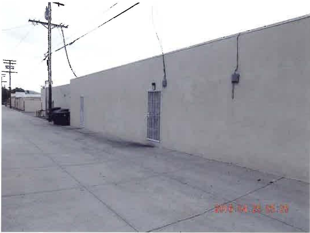
BLDG REAR SIDE, NORTH WALL. From alley.
