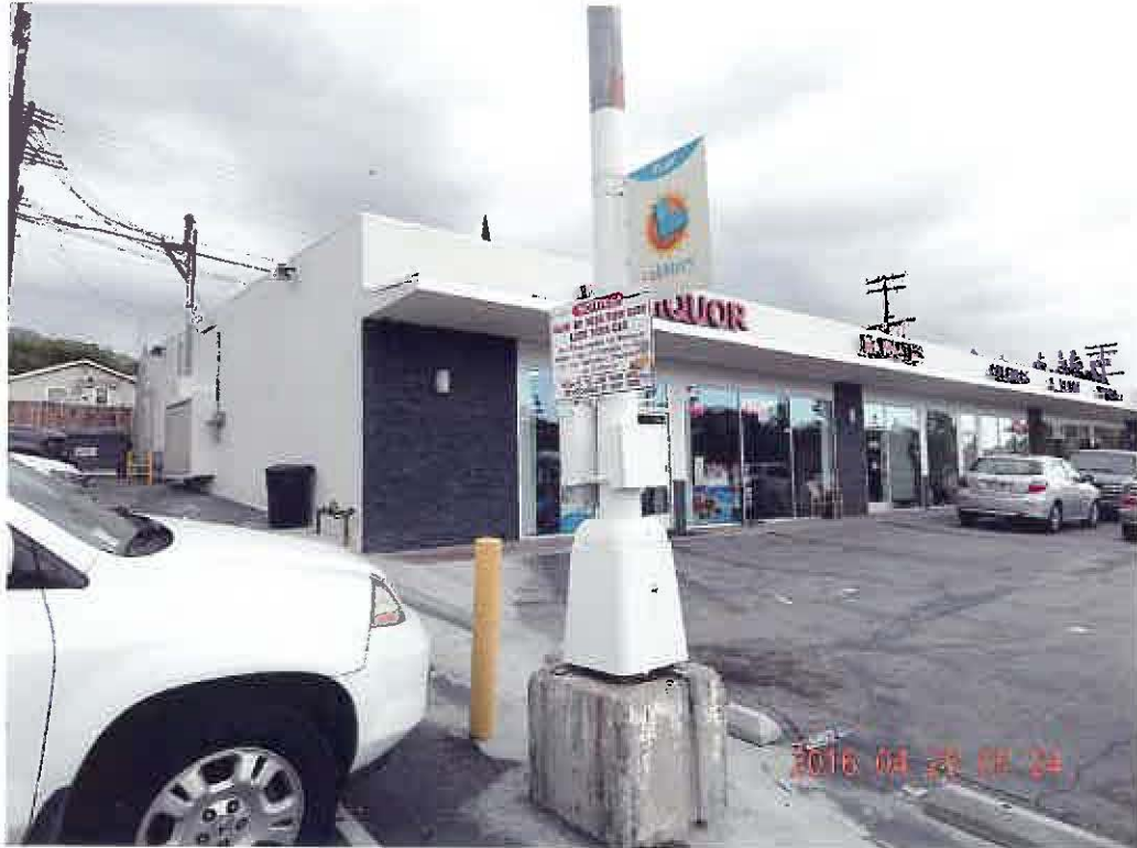
BLDG. SOUTH-WEST CORNER.
