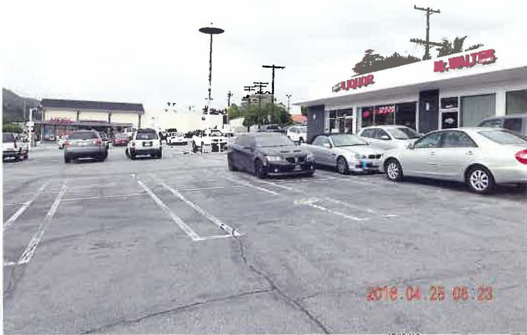
PARKING LOT, west view
