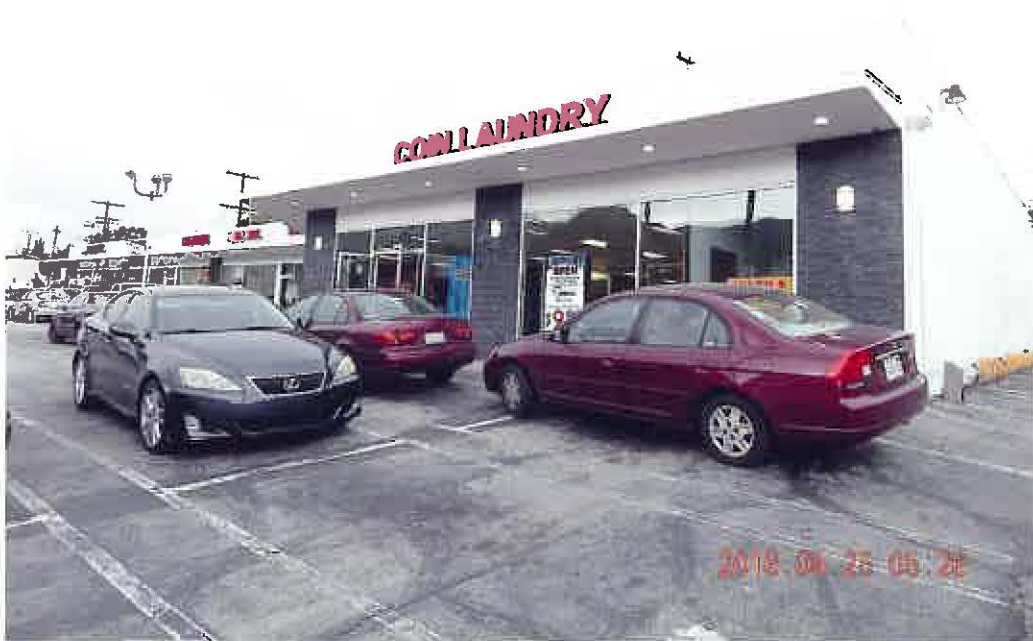
BLDG. SOUTH-EAST CORNER, from side parking.
