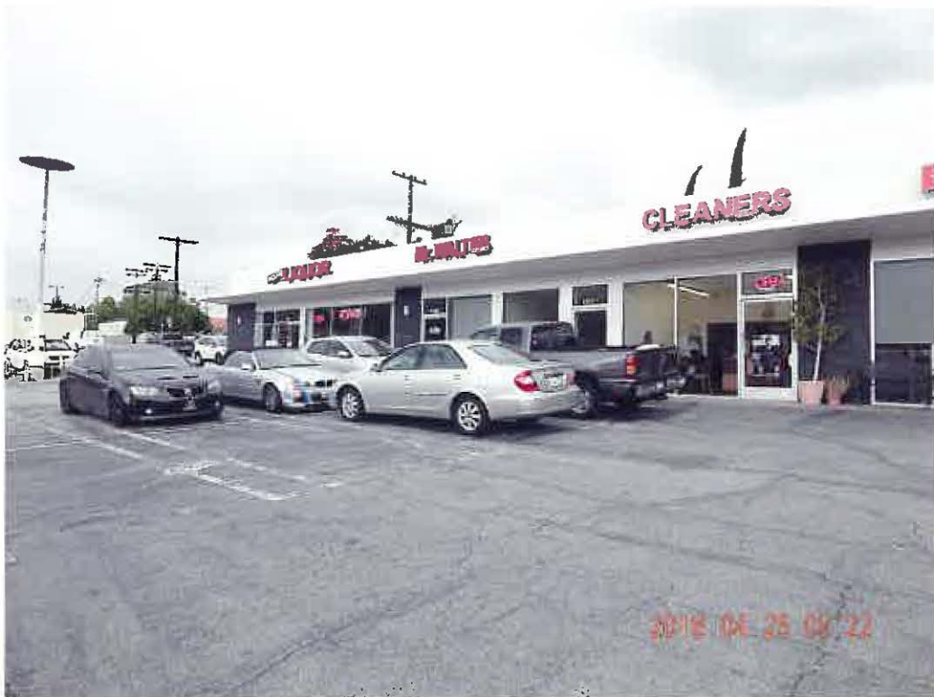
BLDG. SOUTH-WEST CORNER, from parking looking at north-west
