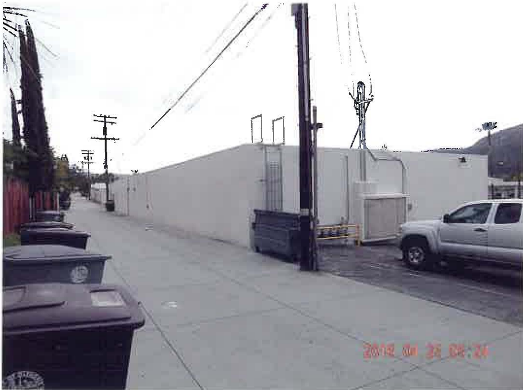
BLDG. NORTH-WEST CORNER, from the alley.
