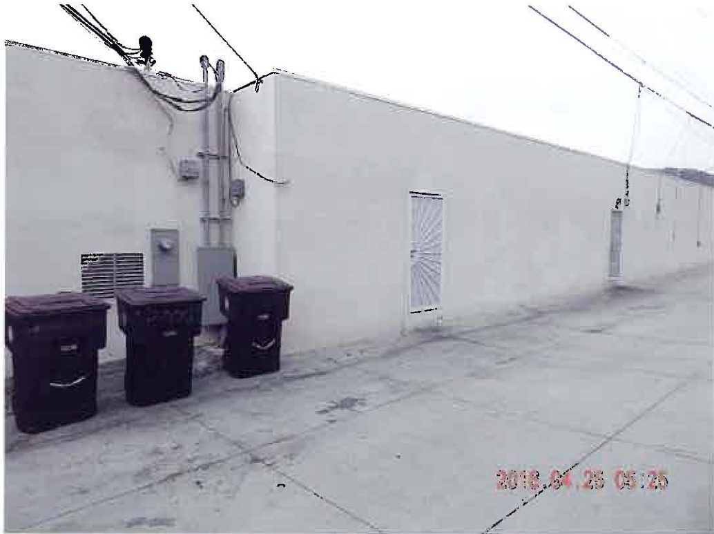
BLDG REAR SIDE, NORTH WALL. From alley.
