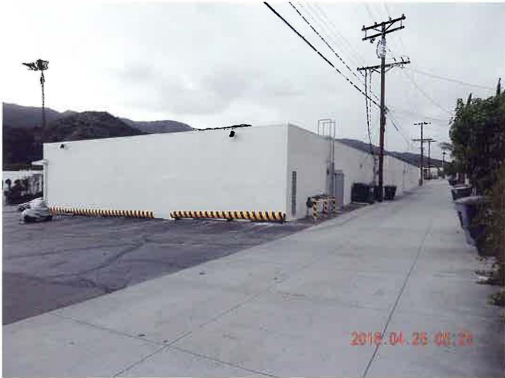
EAST WALL VIEW, from alley.
