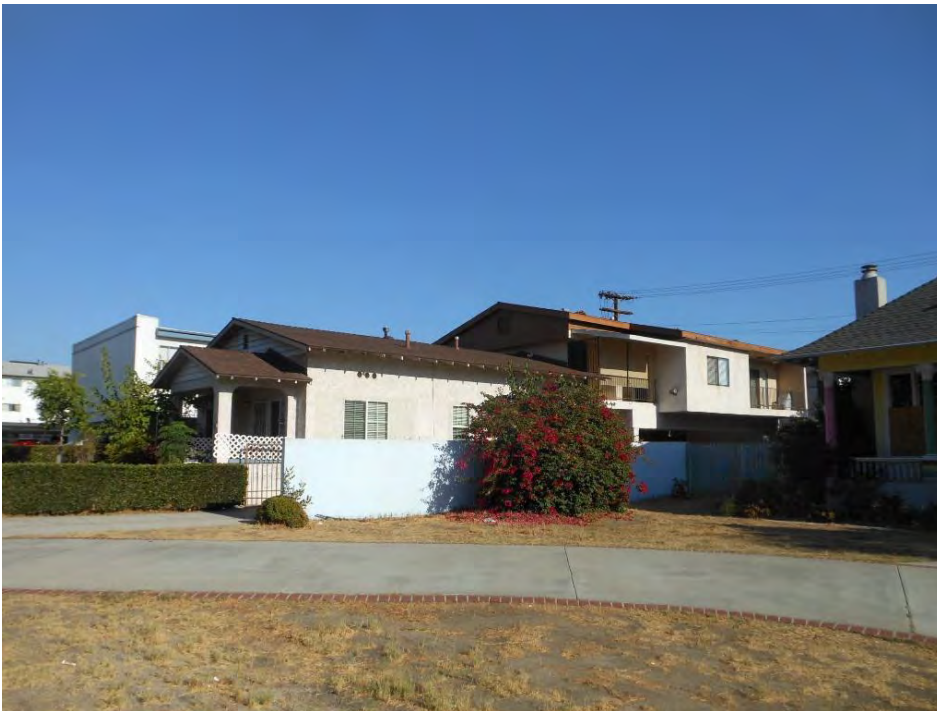
22. 504 West Doran Street, north and west elevations
