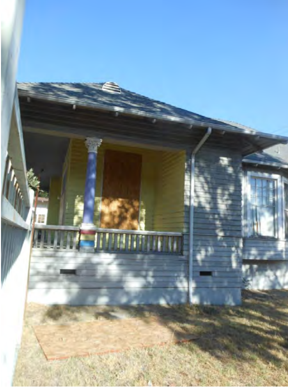
9. 512 West Doran Street, west elevation
