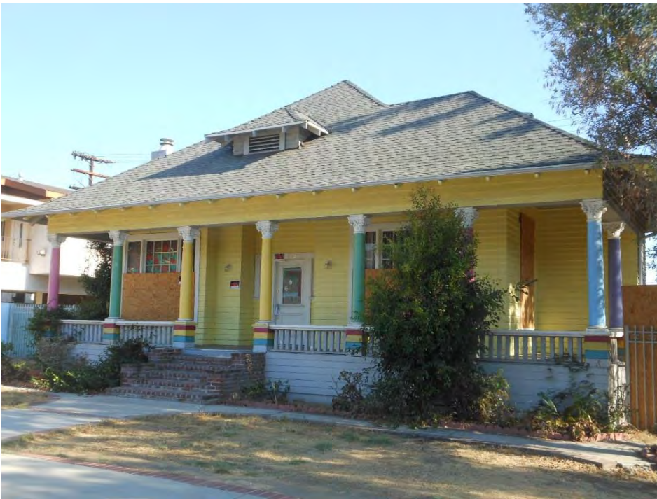
4. 512 West Doran Street, north elevation
