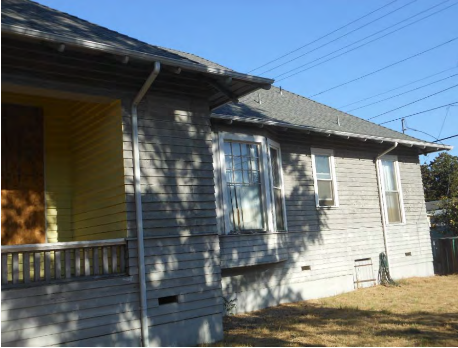
11. 512 West Doran Street, west elevation
