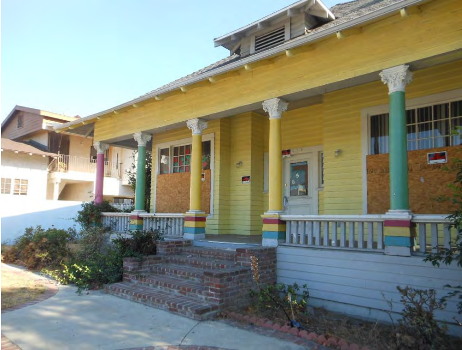
5. 512 West Doran Street, north elevation
