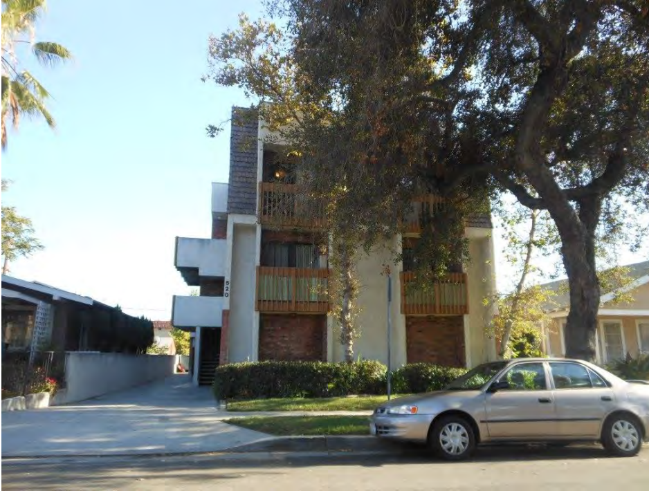
19. 520 West Doran Street, north elevation
