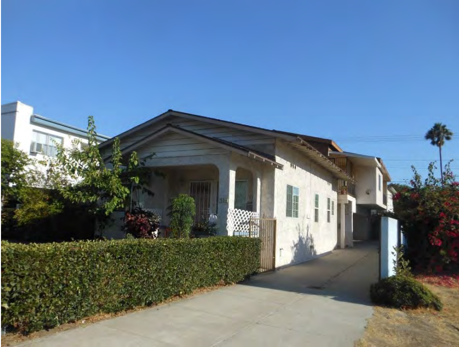
23. 504 West Doran Street, north and west elevations
