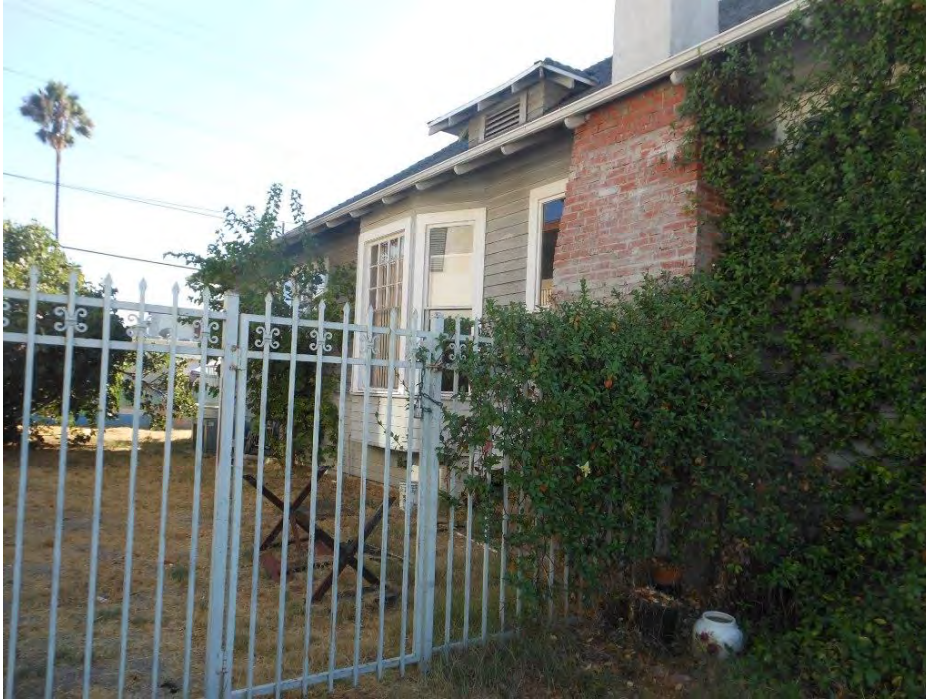
13. 512 West Doran Street, east elevation
