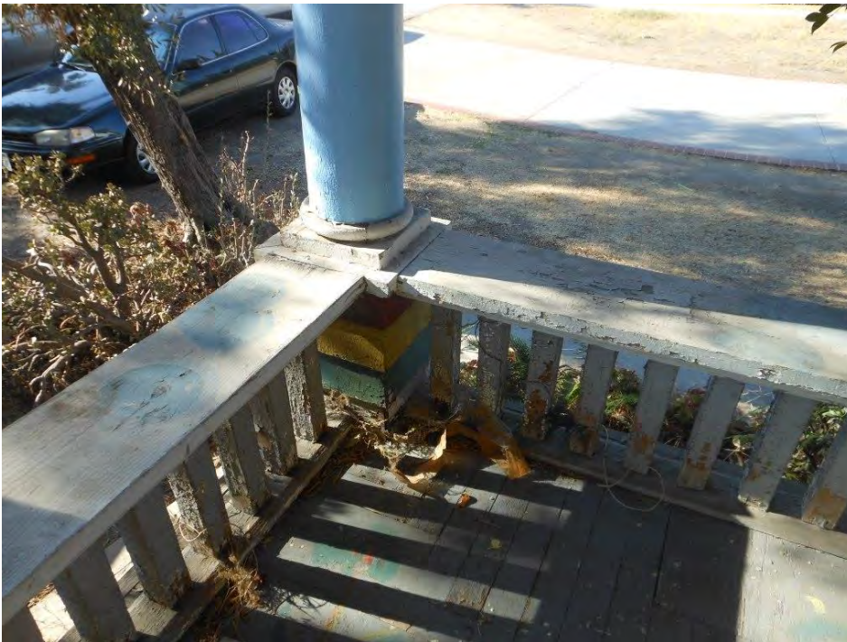
10. 512 West Doran Street, porch detail (656)
