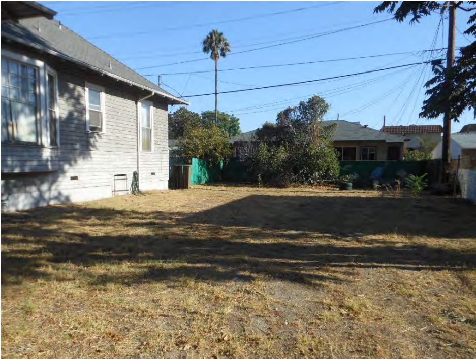
14. 512 West Doran Street, west elevation and undeveloped parcel to west of house
