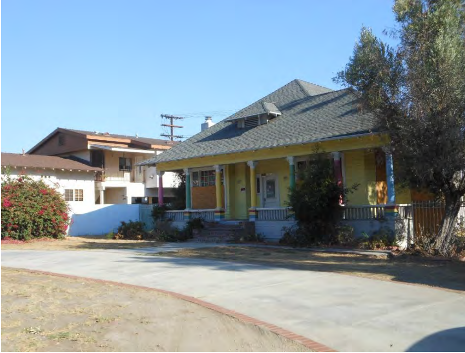
3. 512 West Doran Street, north elevation
