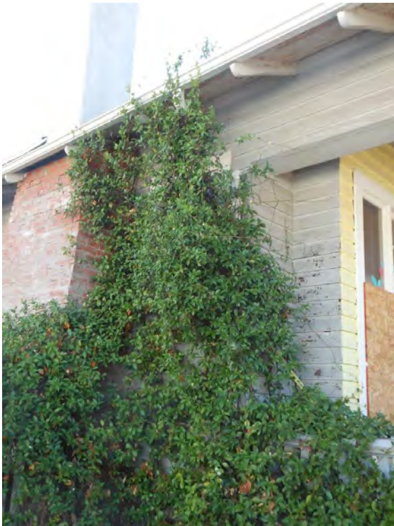
12. 512 West Doran Street, east elevation
