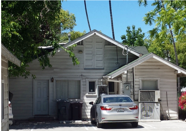
Figure 2. View east of the rear of the house at 128 S. Kenwood, showing hay loft, five-panel doors at the apex of the main gable. The hay loft doors are flanked by decorative attic vents on either side.
