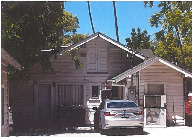
Photograph 1: View east of the rear of the subject property house showing the paired, five-panel hay loft doors at the apex of the main gable. Photograph April 23, 2016.
