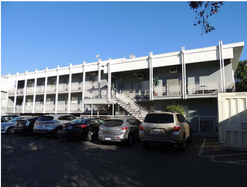
South façade of the apartment building looking north from the neighboring parking lot.
