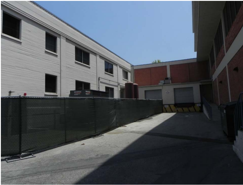
Interstitial space between the 1938 and 1971 buildings looking east from alley.
