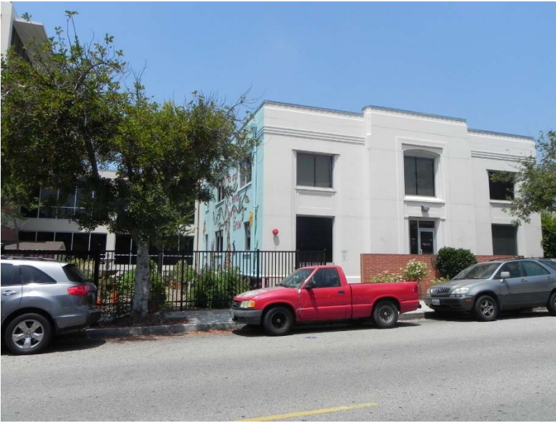
East (primary) façade of the 1938 warehouse building looking west from N. Jackson Street.
