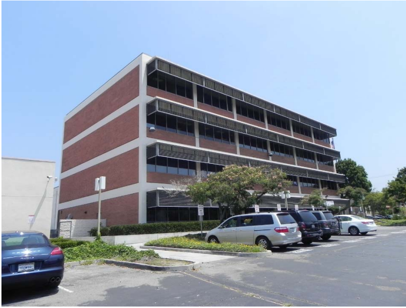
1971 administration building looking northeast from the parking lot.
