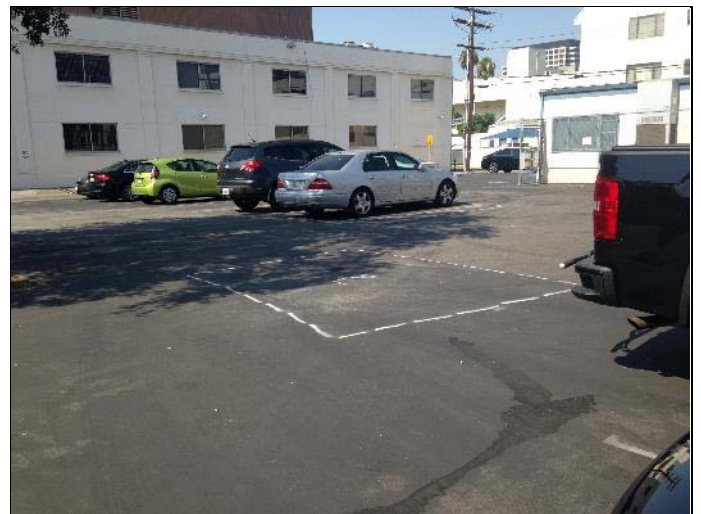
4. View looking southwest across the eastern parking lot toward Building A – modular buildings on right
