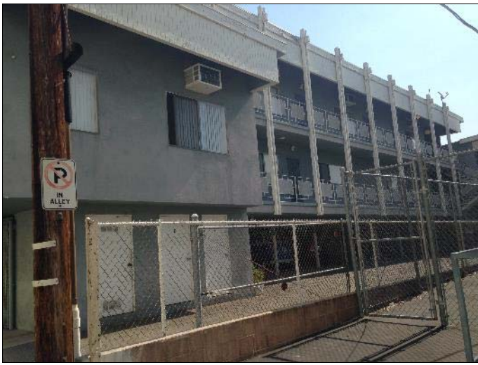
7. View of the south side of the residential apartment building
