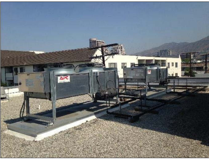
19. View across roof of Building A
