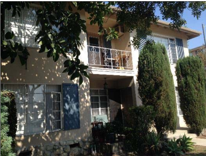
21. View of residential apartment building to the north
