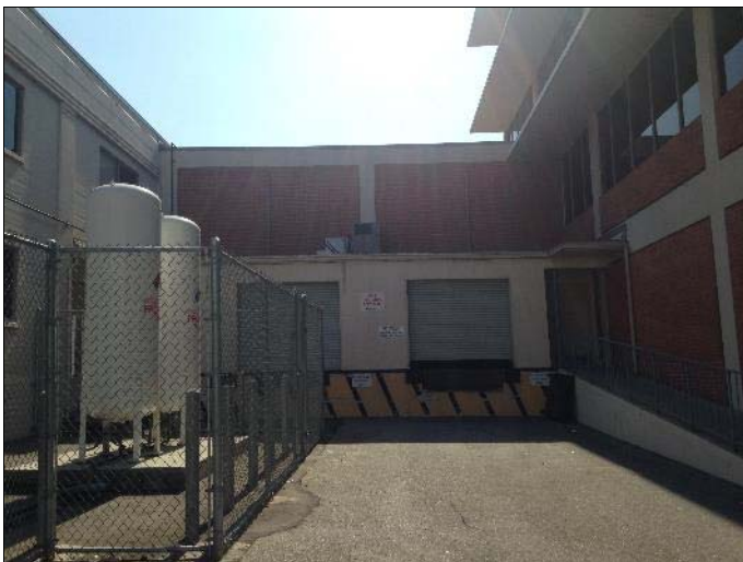
3. View looking east of the loading dock and propane ASTs between Buildings A (left) and B (right)
