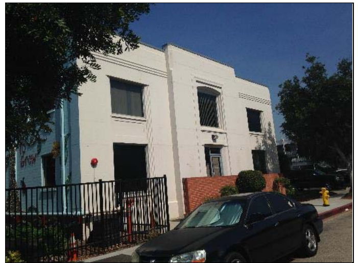
2. View looking northwest of the front entrance to Building A
