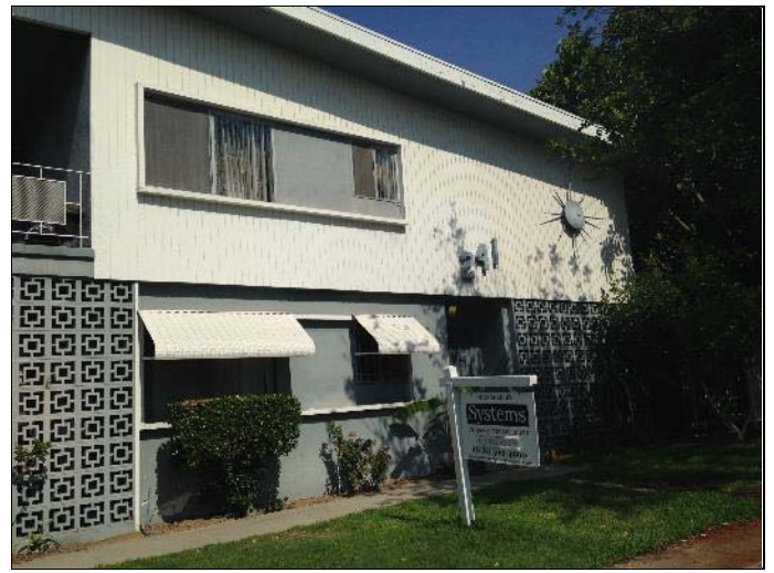
20. View of the front (east) side of the onsite residential apartment building
