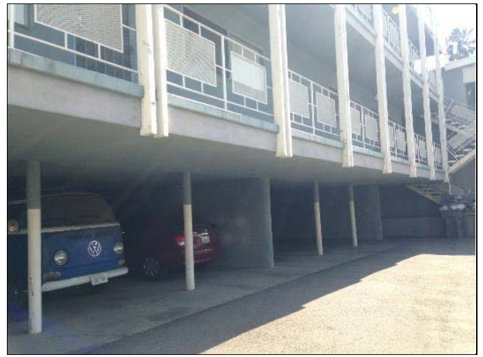
8. Tuck under parking at the residential apartment building
