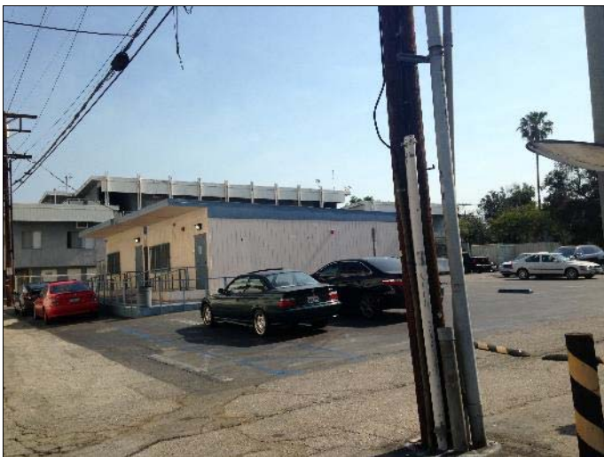
9. View looking north/northeast toward the modular classroom buildings
