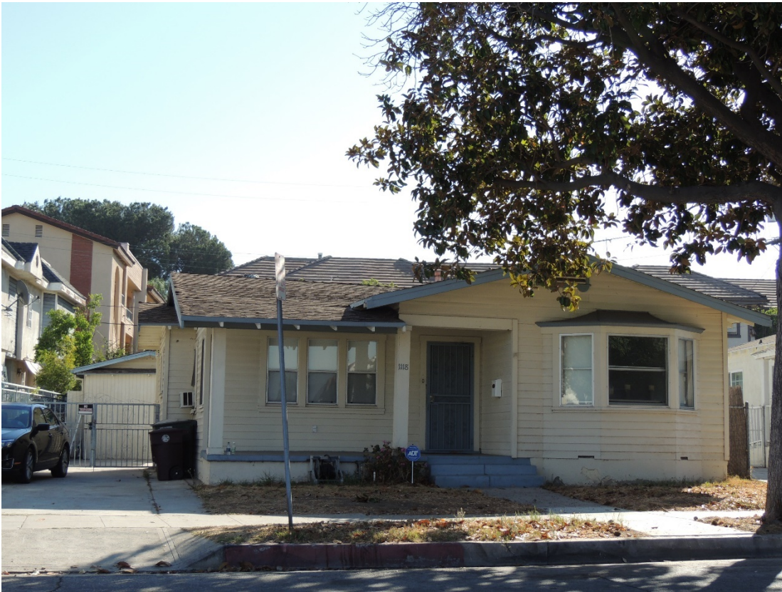
1118 N. Columbus Avenue, view facing southeast.
