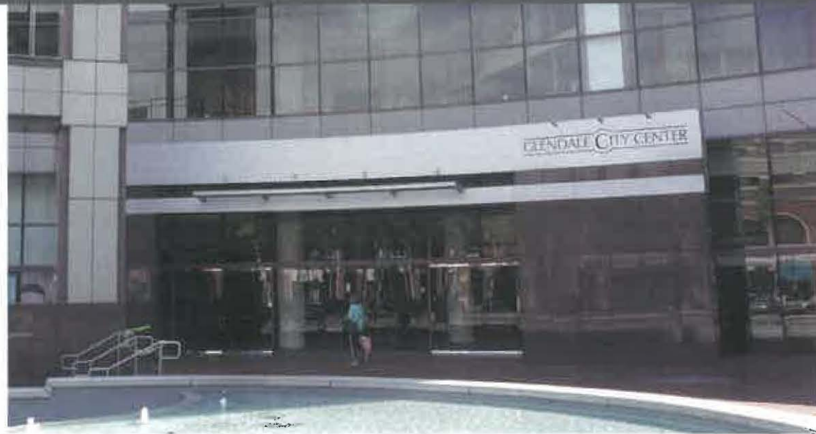
Existing entrance portico with building ID sign
