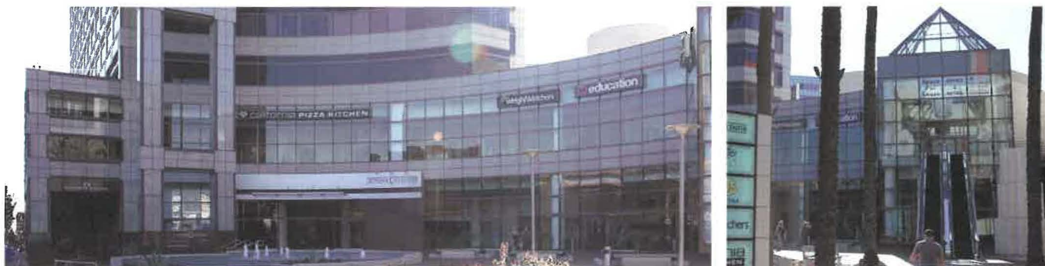
Existing photo of facade/plaza area
