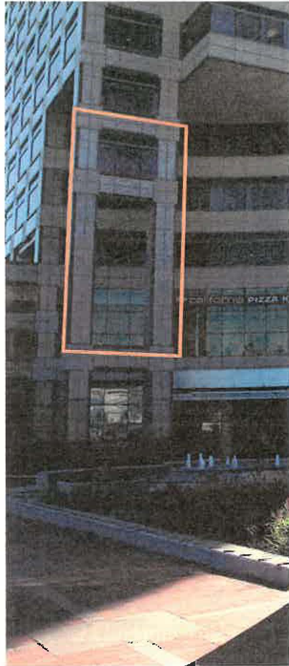
Existing ladder-like structure of the building on North Brand Blvd
