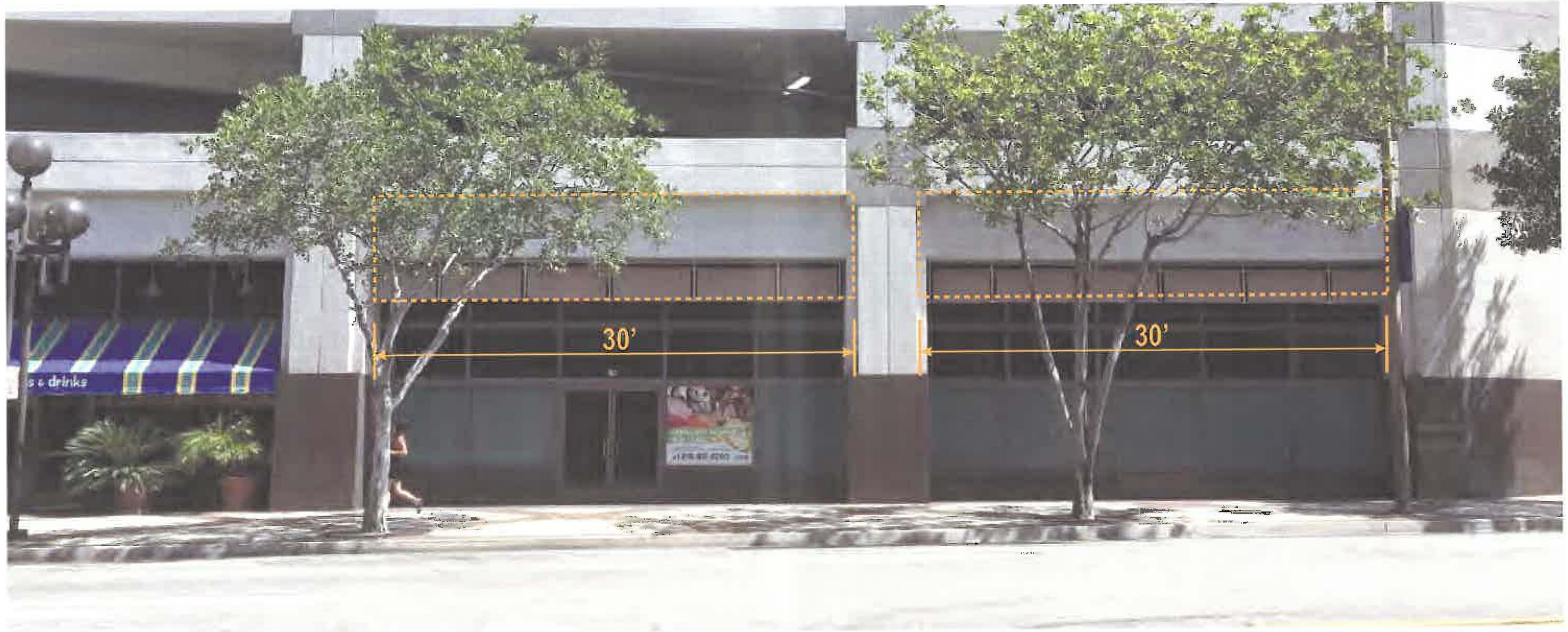
Proposed wall sign location for Suite 180, vacant
