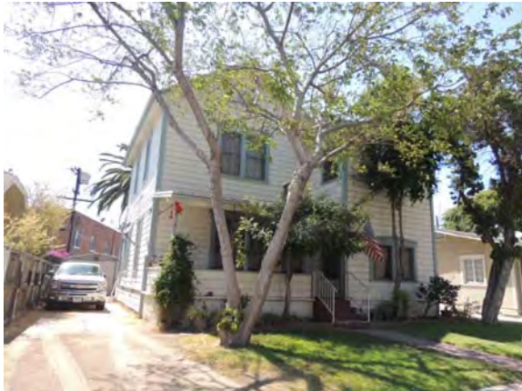
227 Everett St. Source: Historic Resources Group, July 2014.
