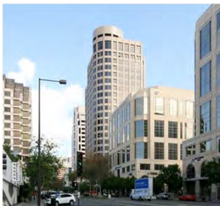
Sears Savings Plaza (1980, Welton Becket and Associates) is an example of the type of high-rise office development that permeated Brand Boulevard in the 1980s and 1990s. Source: http://www.you-are-here.com/modern/sears.html
