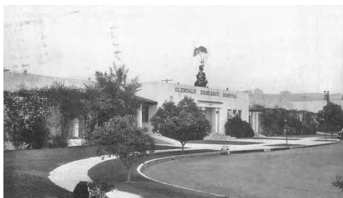
Glendale Research Hospital (1921, Charles W. Kent & Son builders) at N. Adams Street and Doran Drive adjacent to Piedmont Park. The E-shaped plan featured Spanish Colonial Revival pergolas on each side of the main entrance. French doors from all rooms allowed patients to recuperate outdoors. Source: Special Collections Room, Glendale Public Library.
