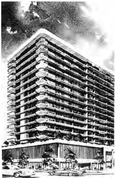
Monterey Island (1983, Krisel/Shapiro & Associates) at 222 Monterey Road. Los Angeles Times , Display Ad 85, May 2, 1983.
