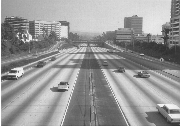
High-rise development lining the 134 Freeway. Source; Special Collections Room, Glendale Public Library.
