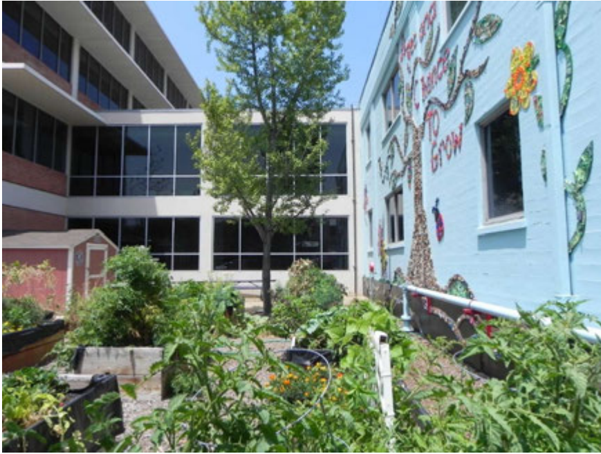
Interstitial space between 1938 and 1971 buildings with connecting hyphen. Looking west from N. Jackson Street.
