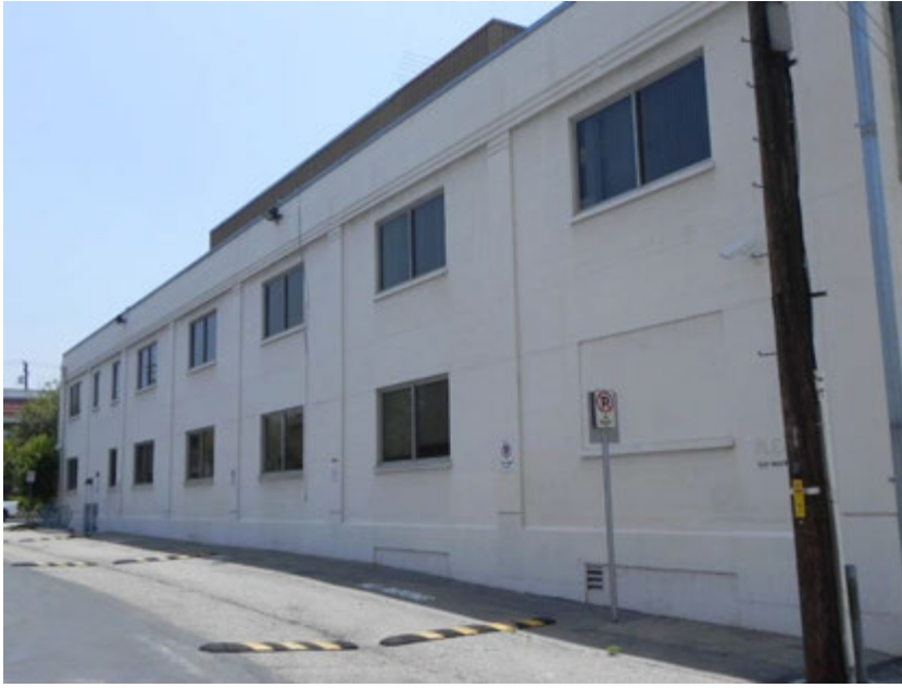
North façade of the 1938 warehouse building looking southeast from alley.
