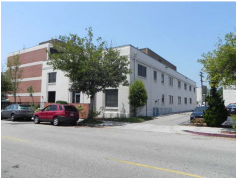
1938 warehouse building looking southwest from N. Jackson Street.
