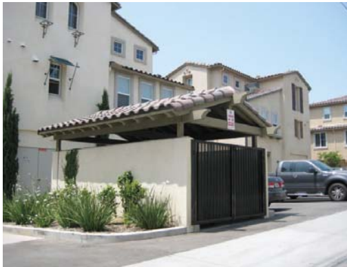
Equipment screening complements building
