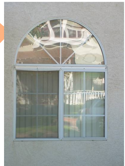
Internal grid does not recall appearance of true divided-light window
