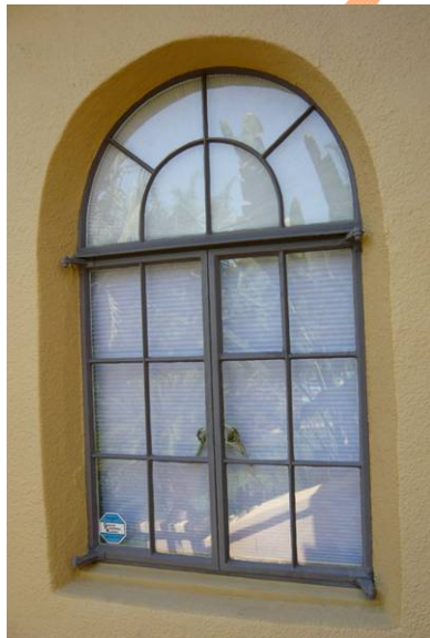
Deep recess with beveled sides and stucco sill
