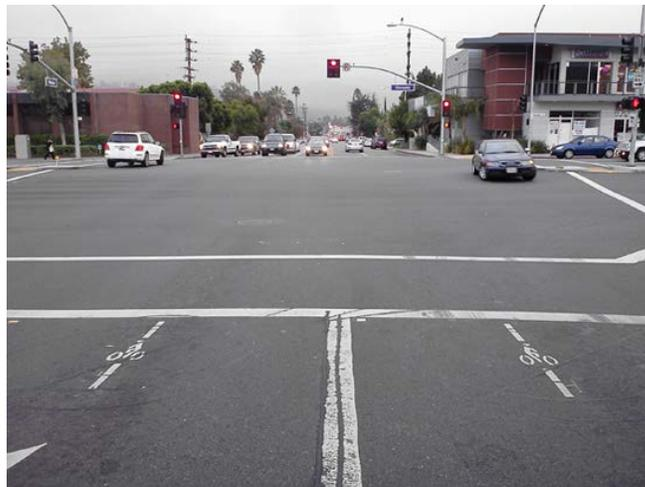
As part of the City's Bicycle Master Plan, Glendale, like several California cities, has been including bicycle detection devices in all traffic signal installations and modification projects. The detection of bicyclists at signalized intersections can improve efficiency, decrease delay to bicyclists, and most importantly, promote safety by assuring that cyclists are provided with sufficient green time to clear the intersections.
