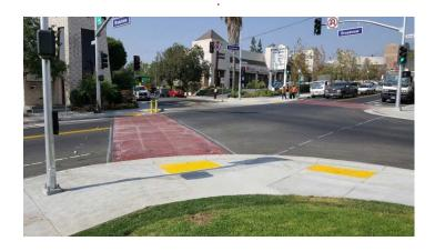
Work on the Ocean View Blvd. Rehabilitation Project is wrapping up! In late September through October, crews removed and installed new pavement, and constructed new stamped concrete crosswalks at the intersections of Ocean View with Broadview and Sunview Drives. This project has made driving, walking, and biking on Ocean View a safer and more pleasant experience for everyone – make sure to visit and check it out soon! More information on the project can be found <u>here</u>.
