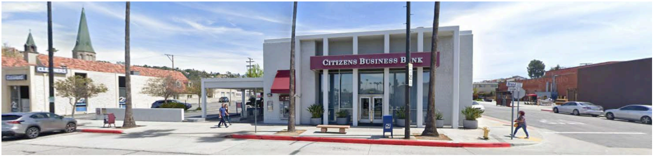
27. 105 E. Glenoaks Blvd: view looking east at the neighboring businesses to the north of the subject property.
