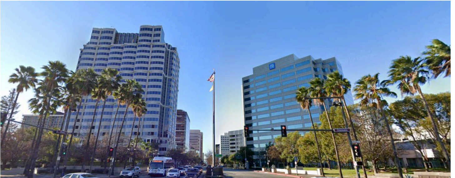
24. 105 E. Glenoaks Blvd: view looking southwest at the neighboring businesses to the southwest of the subject property.
