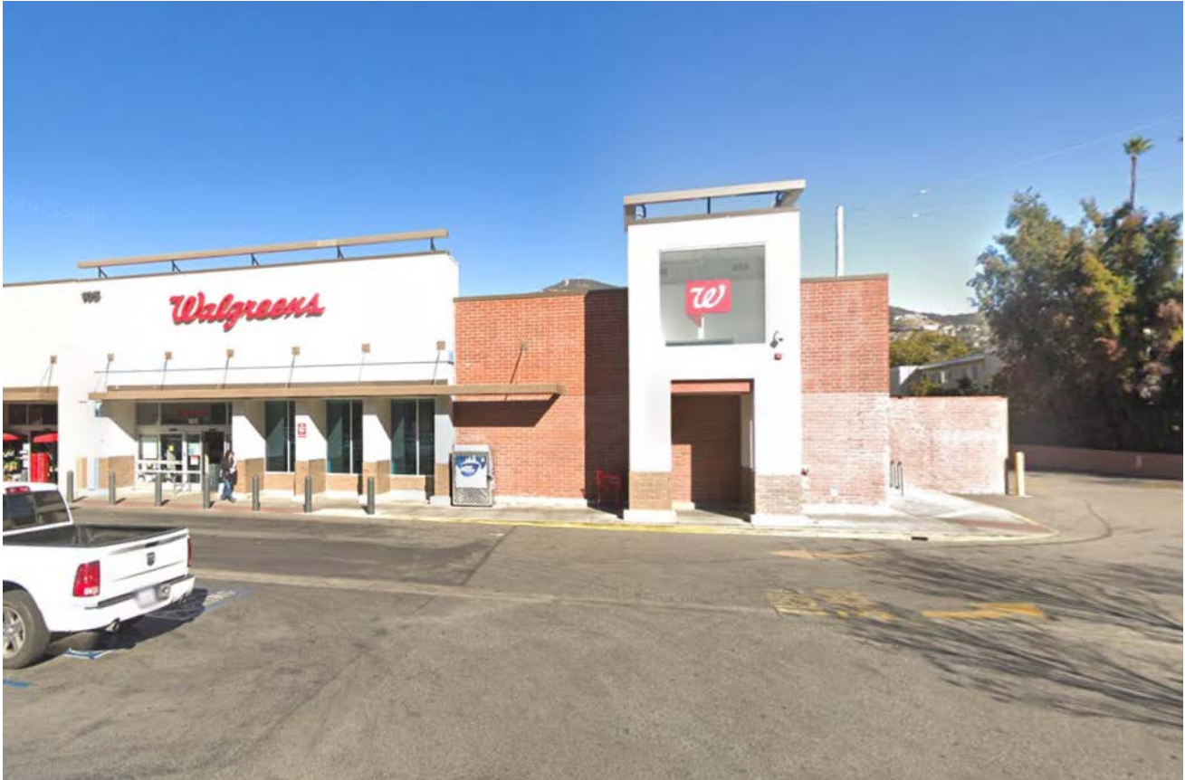
1. 105 E. Glenoaks Blvd: view looking at the front entrance on the south side of the subject property.
