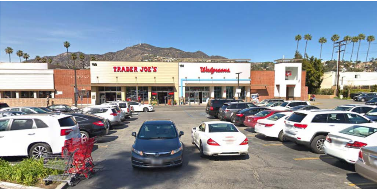
2. 105 E. Glenoaks Blvd: view looking north at the south side of the subject property.
