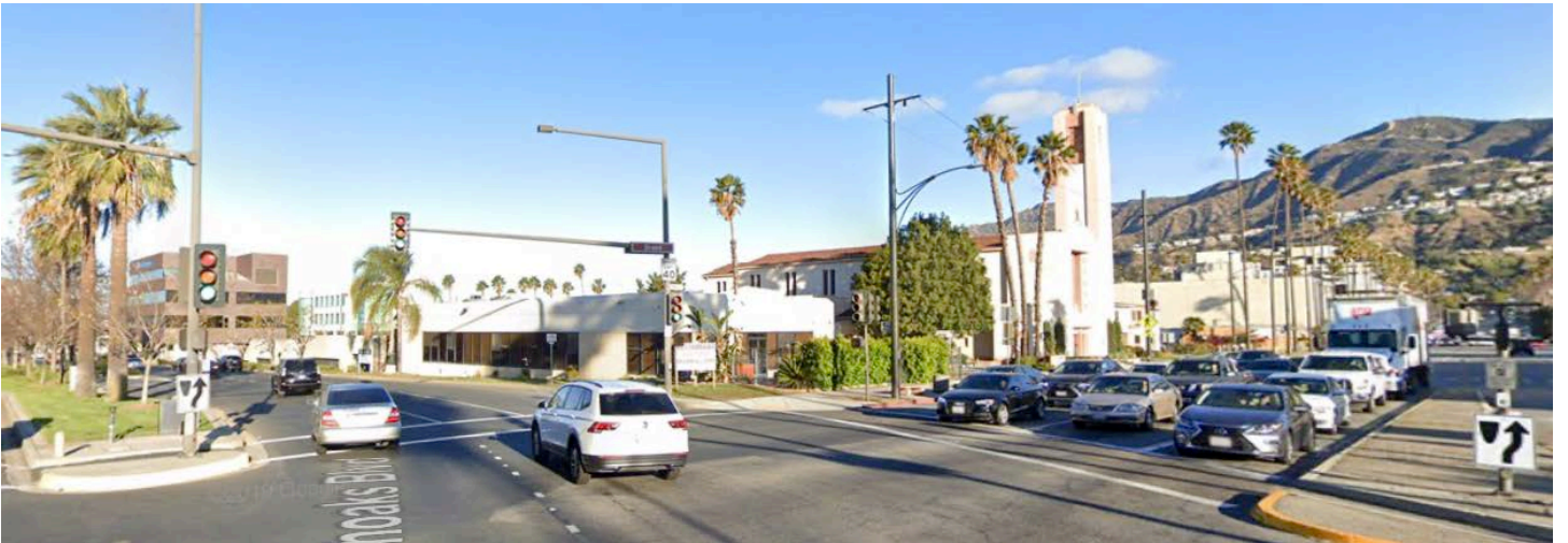
25. 105 E. Glenoaks Blvd: view looking west at the neighboring businesses to the west of the subject property.
