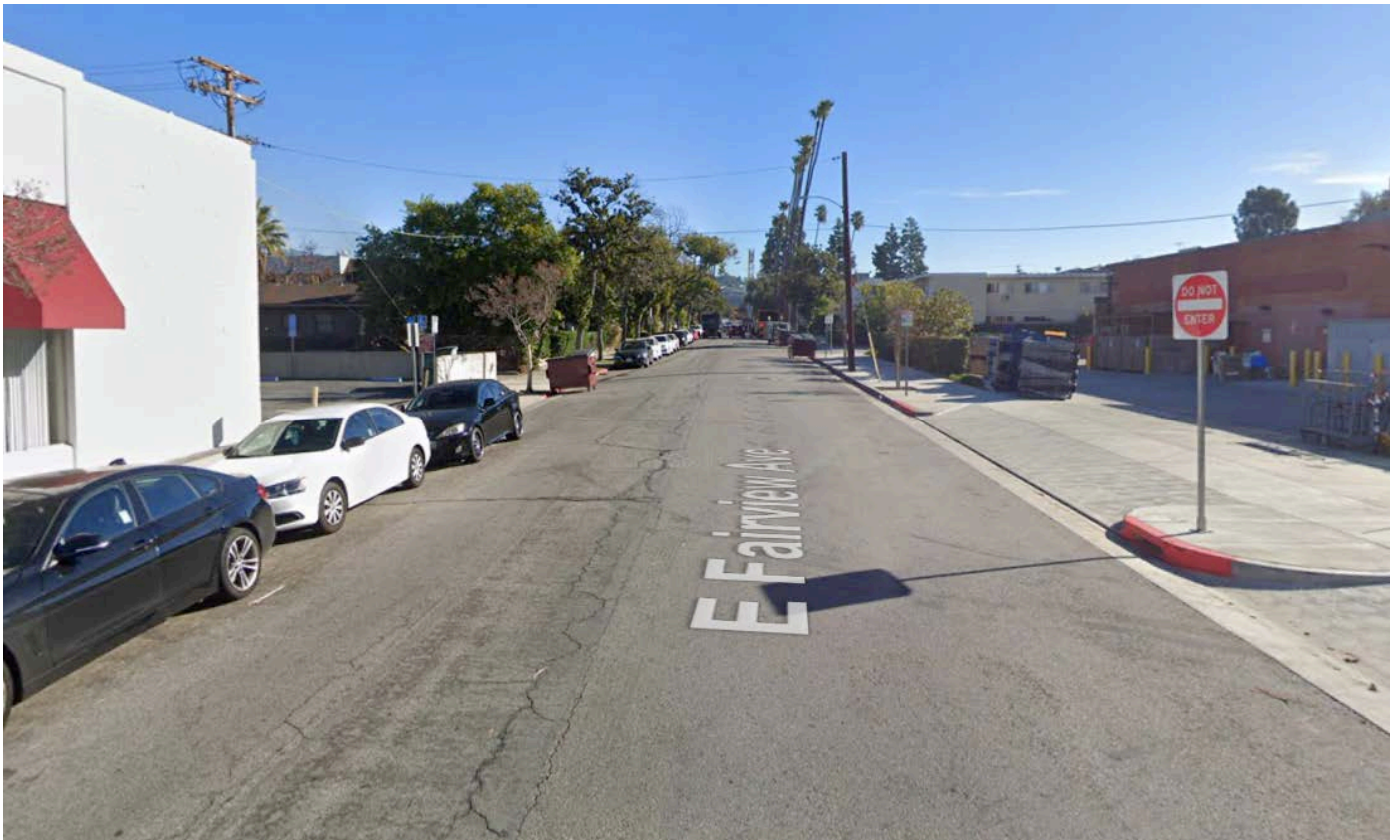
21. 105 E. Glenoaks Blvd: view looking east along E. Fairway Ave. to the north of the subject property.
