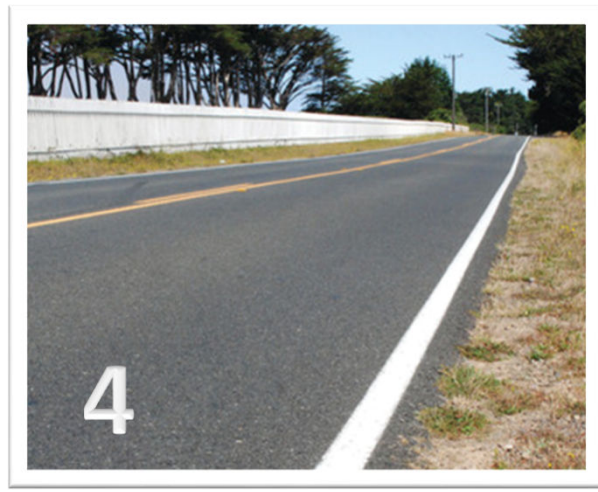
Striping and Marking
