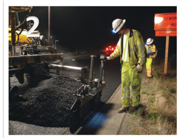
Installation of A.R.H.M.
