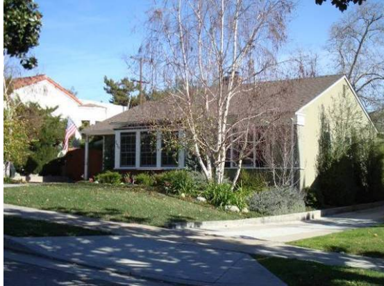
Well-crafted windows provide quality details for simple buildings
