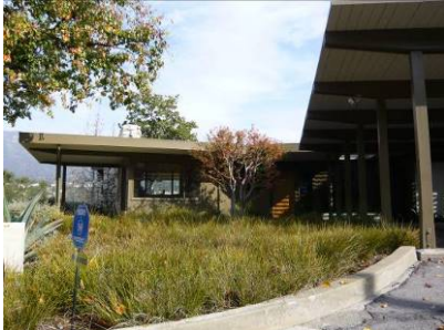
Strong architectural idea: post and beam “L” shaped house with extended eaves
