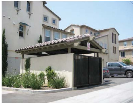
Equipment screening complements building
