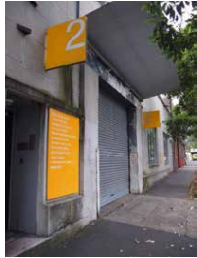
Industrial Design Studio Retrofit Sydney, Australia
