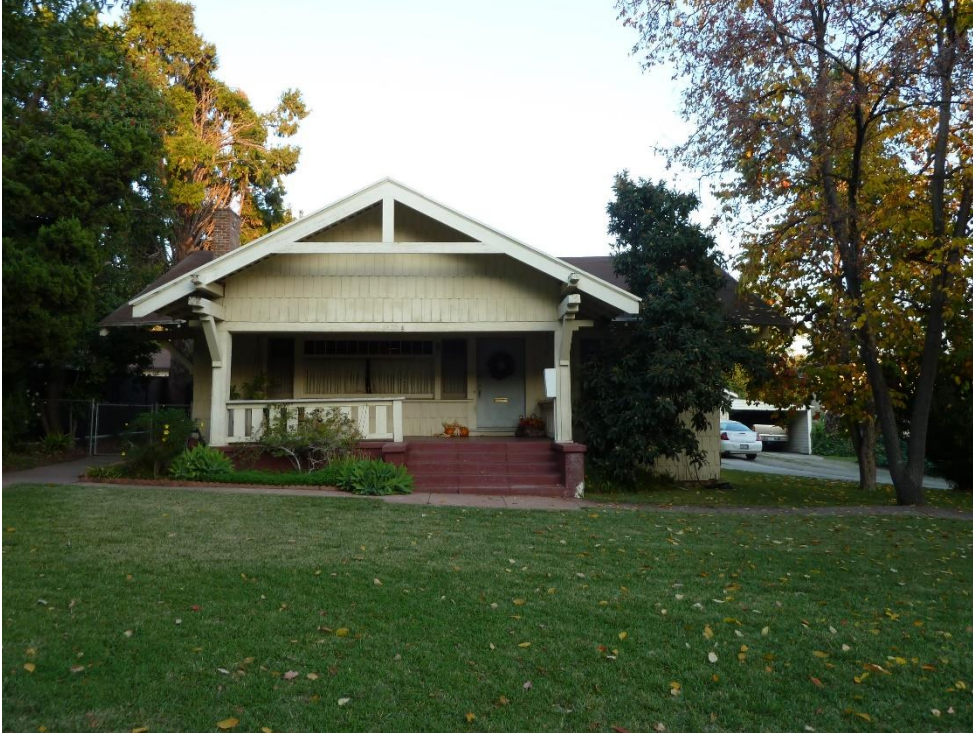
Figure 3.2-2. 1420 Valley View Road, View of Primary (west) Elevation of the Residence
