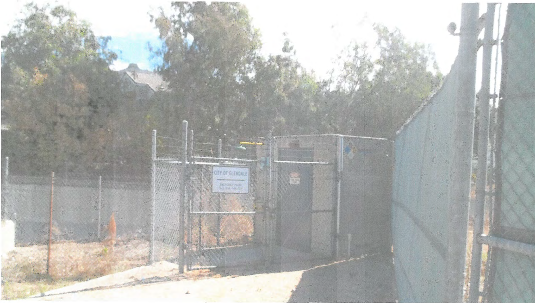
GWP Chlorination Station
