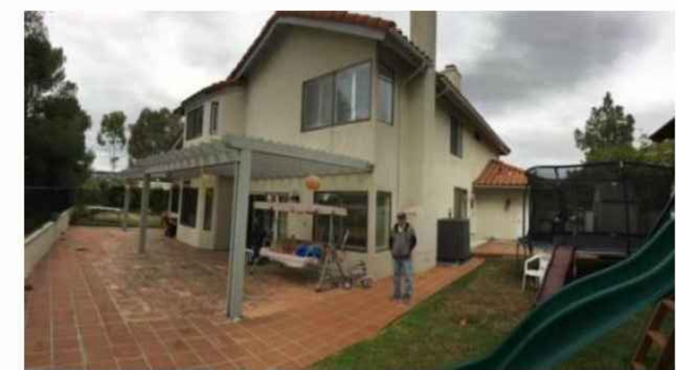
REAR SIDE CORNER
