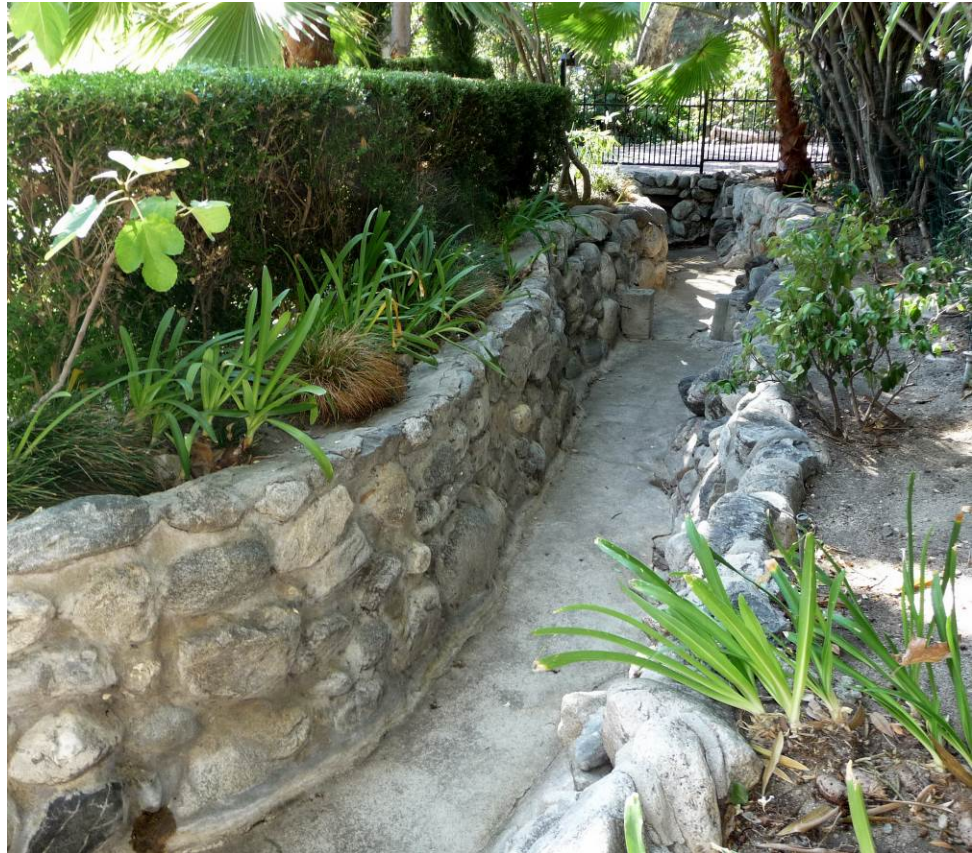
Figure 27. Stone stream bed on the east side of Niodrara Drive, passing through the 1808 Niodrara Drive property. Photo by ARG.
