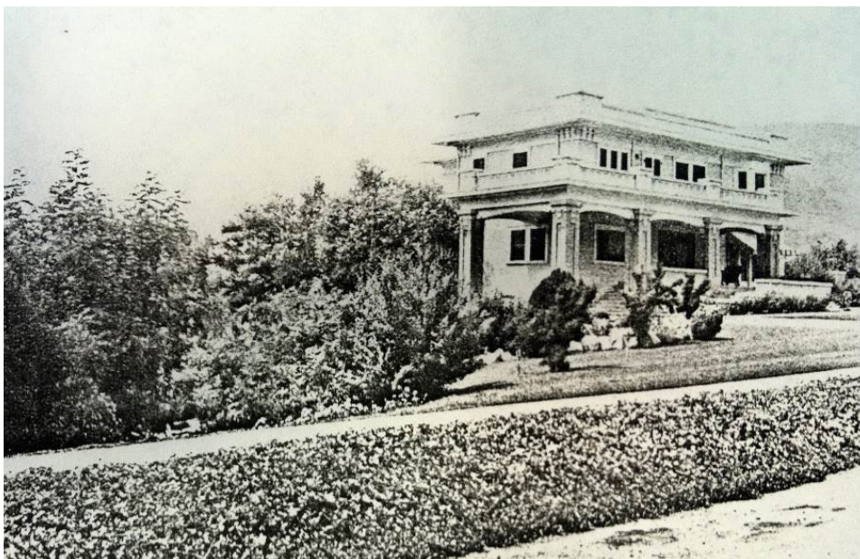
Figure 21. Residence at 1616 Wabasso Way. The earliest house in the subdivision, its site incorporated existing natural features per McLaren’s landscape plan. Source: Glendale Public Library, Glendale Special Collections.
