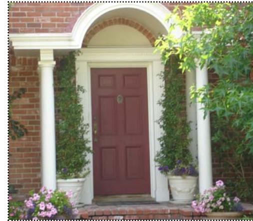
Above: The portico for this Colonial Revival house uses classical elements in its design.
