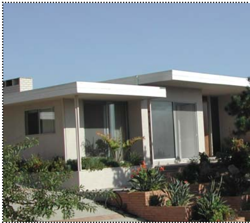
Above: A flat roof is the the most common roof form among Modern styles.
