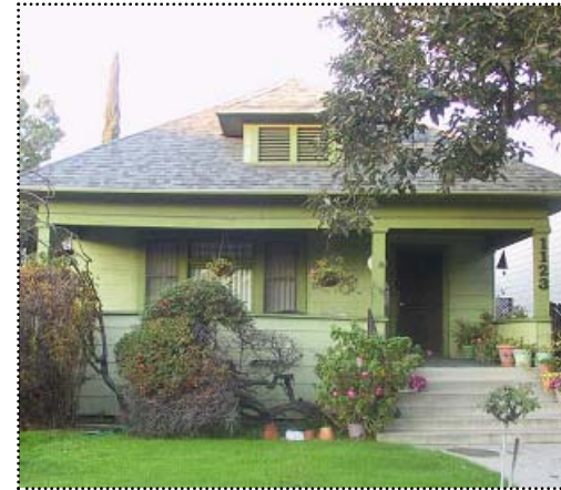
Above: This Queen Anne cottage has narrow wood clapboard siding.
