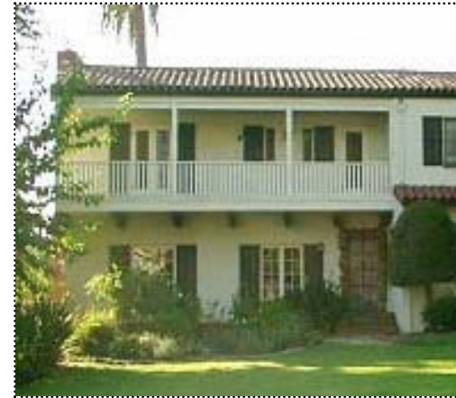
Above: The recessed balcony on the main facade is the primary character-defining feature of the Monterey Revival style.
