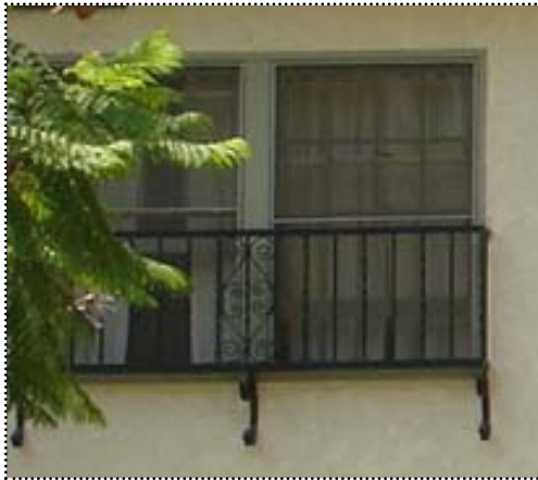
Above: Windows often have decorative wrought iron balconets.
