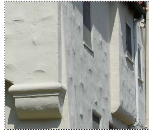
Above: Stucco finish used here is smooth but there are decorative raised areas.
