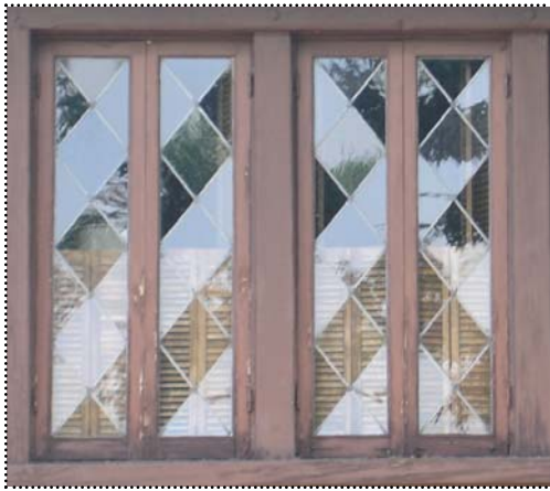
Above: These leaded casement windows are a very important component of the front facade of this house.
