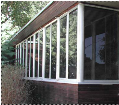
Above: Both the metal casements and the horizontal banding of these windows are characteristic of Modernism.
