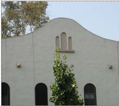
Above: This building has arched windows arranged in pairs and groups of three.
