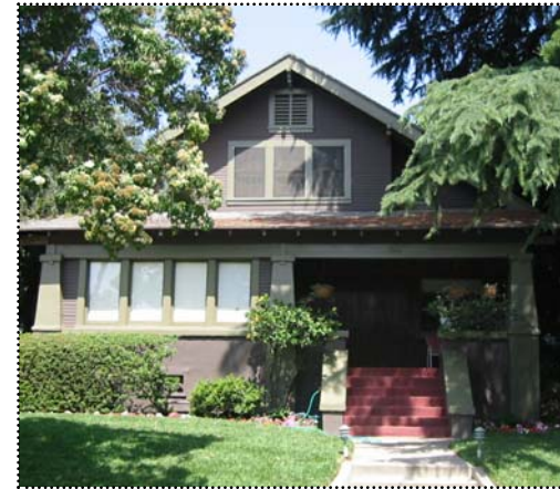
Above: Most Craftsman houses have a forward-facing, prominent gabled roof.
