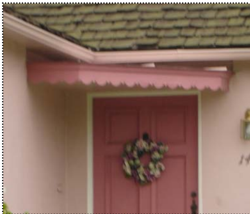
Below: A simple metal canopy with characteristic scalloped edges provides the only shelter to the front door of this Minimal Traditional home.
