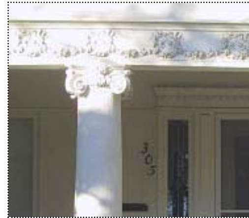
Above: Sometimes ornate classical elements are used in the Mediterranean Revival style.
