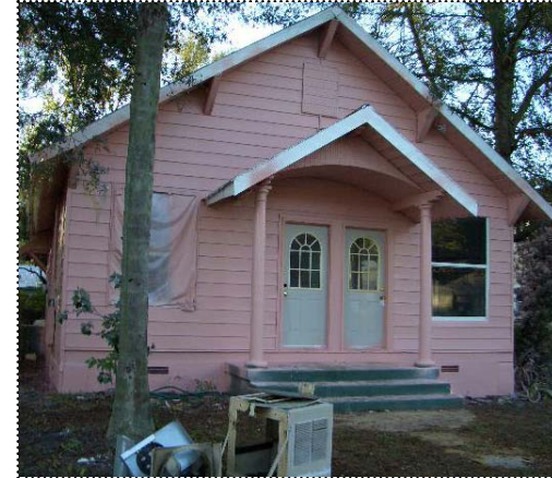
Above: New windows, new doors, poor wood shingle repairs and new stairs would preclude this building from being considered a historic district contributor.
