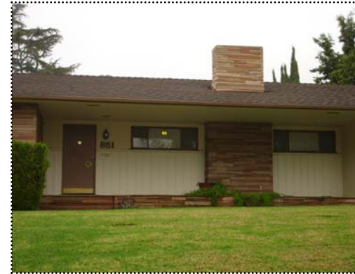
Above: The porch on this house is simply recessed beneath the primary roof. The walkway and the chimney are clad with flagstone.
