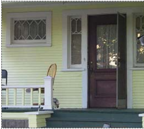
Above: The doors and windows of this house have the simple flat surround characteristic of later examples of the Victorian style. The windows also have stylized muntins.
