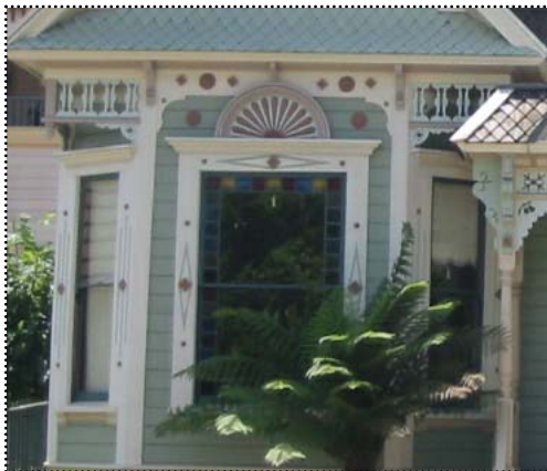
Below: Bay windows are common in more ornate examples of the style.
