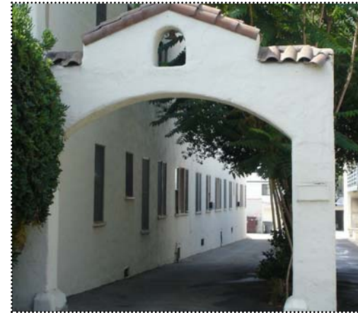
Above: The addition for the driveway appropriately takes the form of the Mission Revival style.
