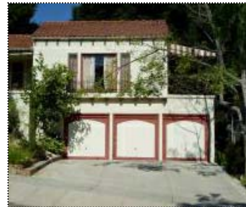
Below: Alterations at the garage level and to the second-story windows impair the integrity of the hillside home.
