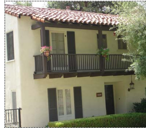
Above: Smooth stucco cladding is a common attribute of the Monterey style.
