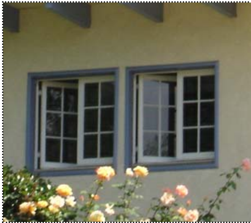
Above: This house has wooden casement windows.
