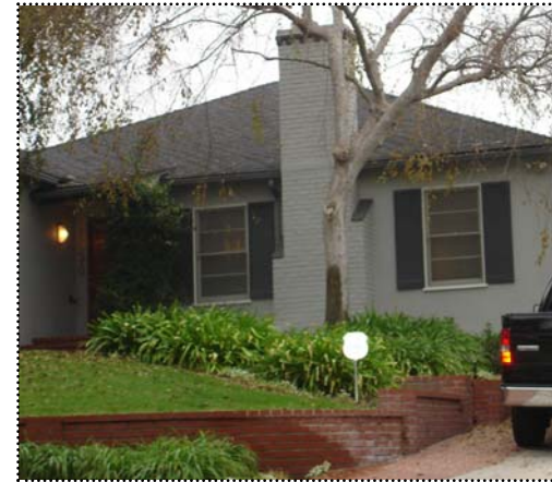
Above: This Minimal Traditional house has a typical stucco exterior.
