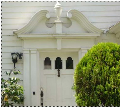
Above: The broken pediment is one of the architectural ornaments that can be found above doors and windows.
