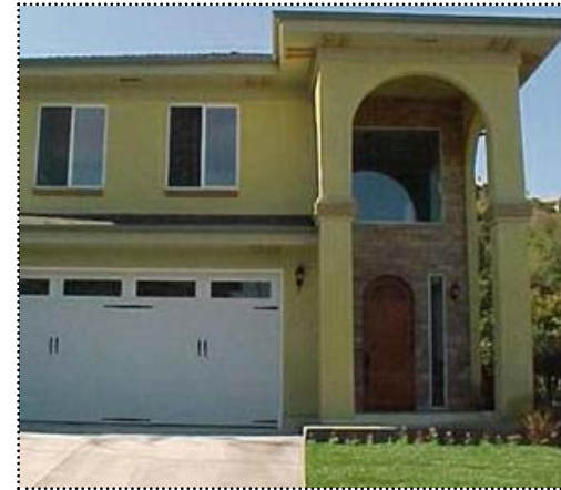
Above: This house was once a split level home from the late 1940s. It has been extensively remodeled and it was constructed outside the period of significance for the surrounding historic district.
