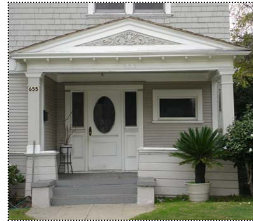
Above: Classically-inspired porch details on this house include a pedimented gable and fluted pilasters with capitals.
