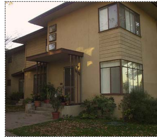
Above: This apartment building, while traditional in form, exhibits the influence of Modernism in its steel casement windows and its clean lines.
