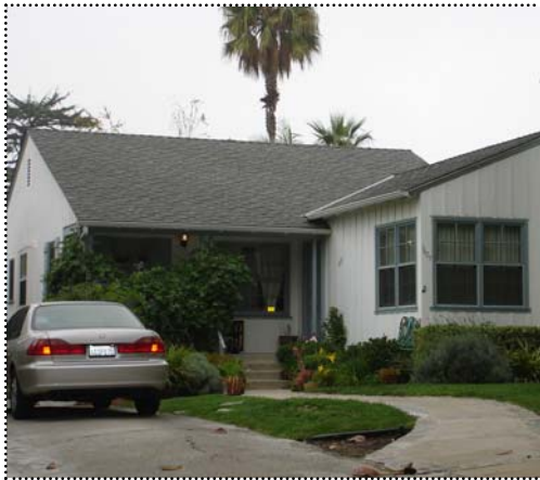
Above: This roof has a primary side gable with a prominent front-facing cross gable.
