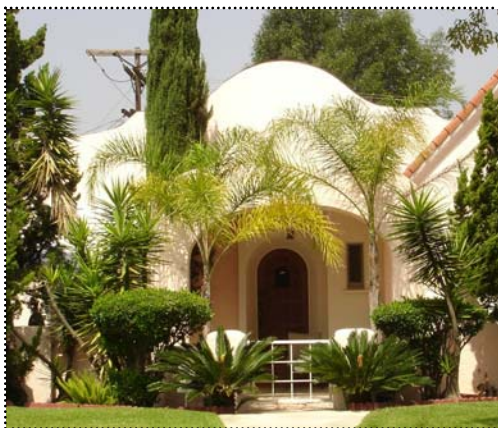
Below: The parapet for this house incorporates the porch with its smooth siding.
