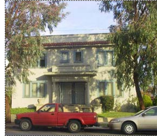
Above: This apartment building has Mediterranean Revival elements including the classical porch and red tile coping at the cornice.
