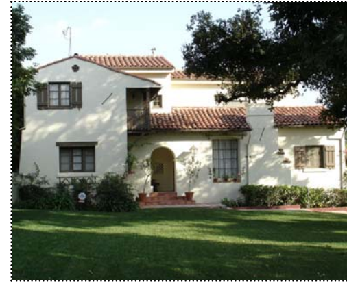
Above: Many period revival style houses, particularly Spanish Colonial Revival style, have a hand-troweled stucco finish that may be either smooth or lightly textured.
