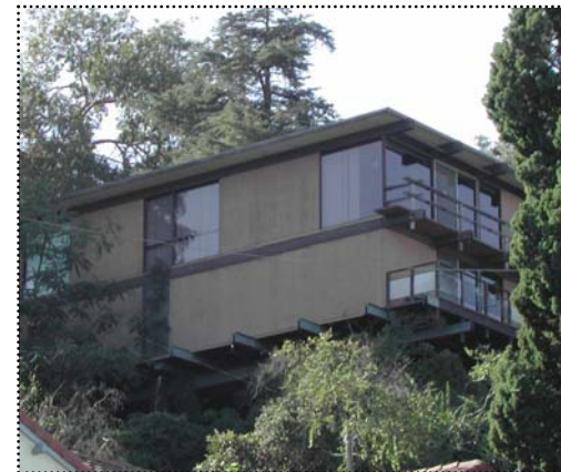
Below: The seamless combination of materials—stucco, wood, and glass—create the smooth and linear character of the exterior walls of this hillside house.
