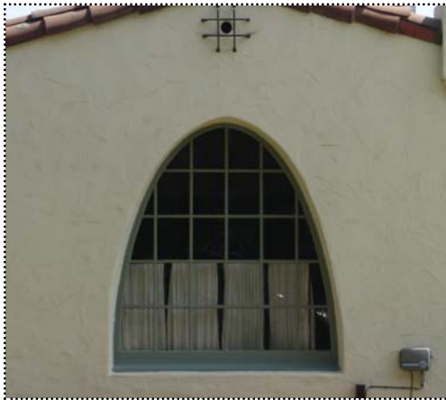
Above: This window has an arched shape that is commonly used in the Spanish revival style.
