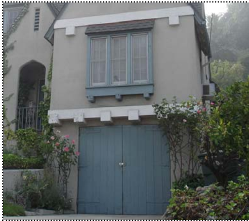
Above: A one-car garage is incorporated on the ground floor of this hillside home. Hillside houses located on the upslope often locate two-car garages in a similar way.
