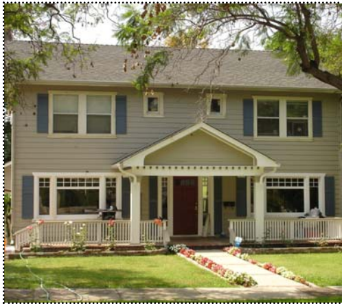
Above: This side-gable roof is the most common roof type of the style in Glendale.
