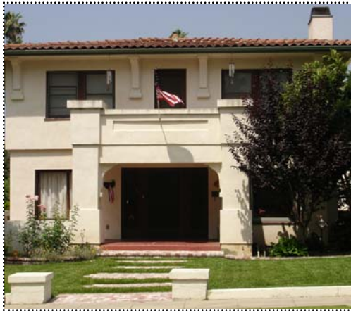
Above: The roof on this house has red tiles. When roof work is required, clay tiles should be removed, cleaned and re-installed.
