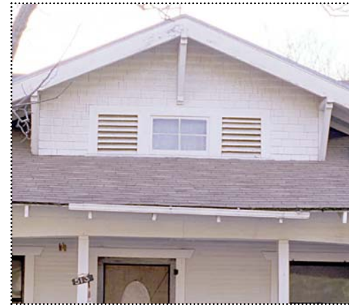
Above: This dormer has simple attic grilles and roof brackets that provide visual interest to the house.
