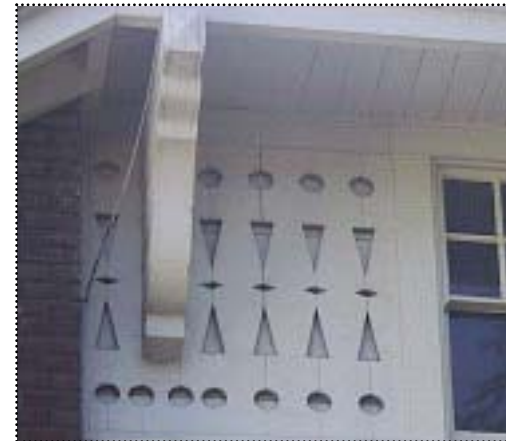
Above: Decorative woodwork in the gable peak is characteristic of the Victorian style.
