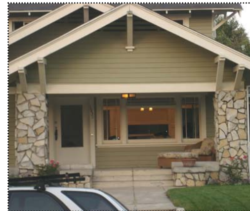
Below: The flagstone supports of this porch are inappropriate to the Craftsman style and should be replaced with its original materials.
