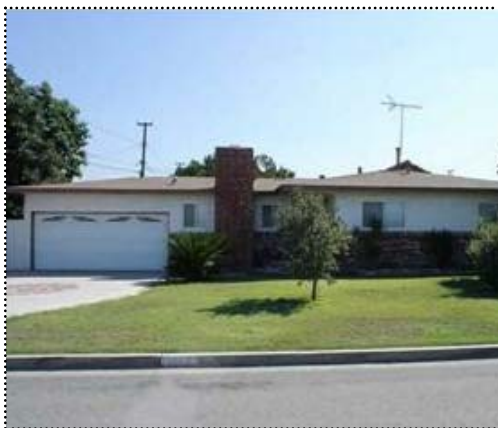
Below: This Ranch style house has new windows and new vinyl siding. It is a non-contributing house in a district of Spanish eclectic bungalows.
