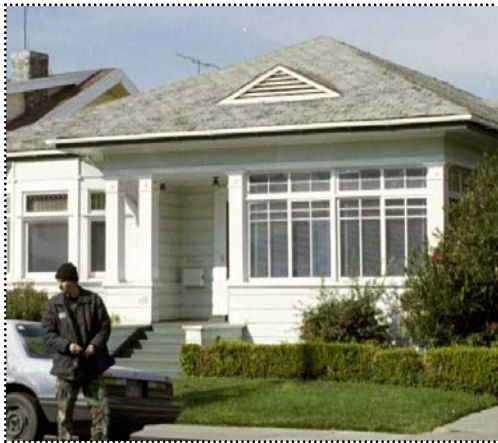
Above: In some cases, the use of glazing can be an appropriate design solution for enclosing a historic porch.
