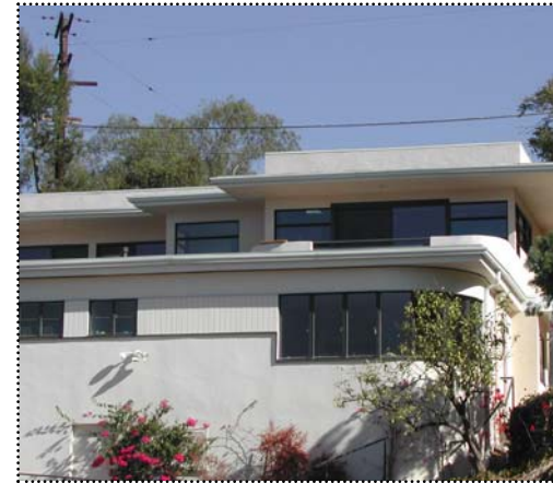
Above: Stucco finishes like this one are common in Modern styles.
