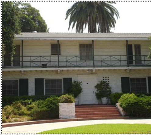
Above: The eave for this roof provides little overhang. The roof cladding is composition shingle.
