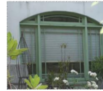
Below: This arched window provides a focal point to the facade. There are both fixed and operable components to the window.
