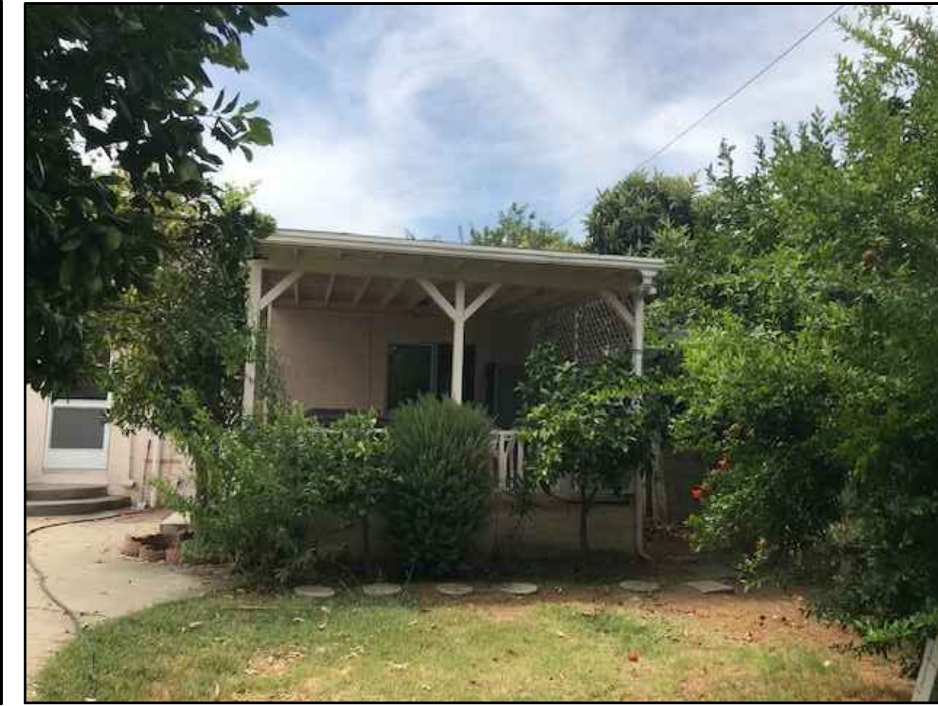
NORTH ELEVATION (partial rear view)
