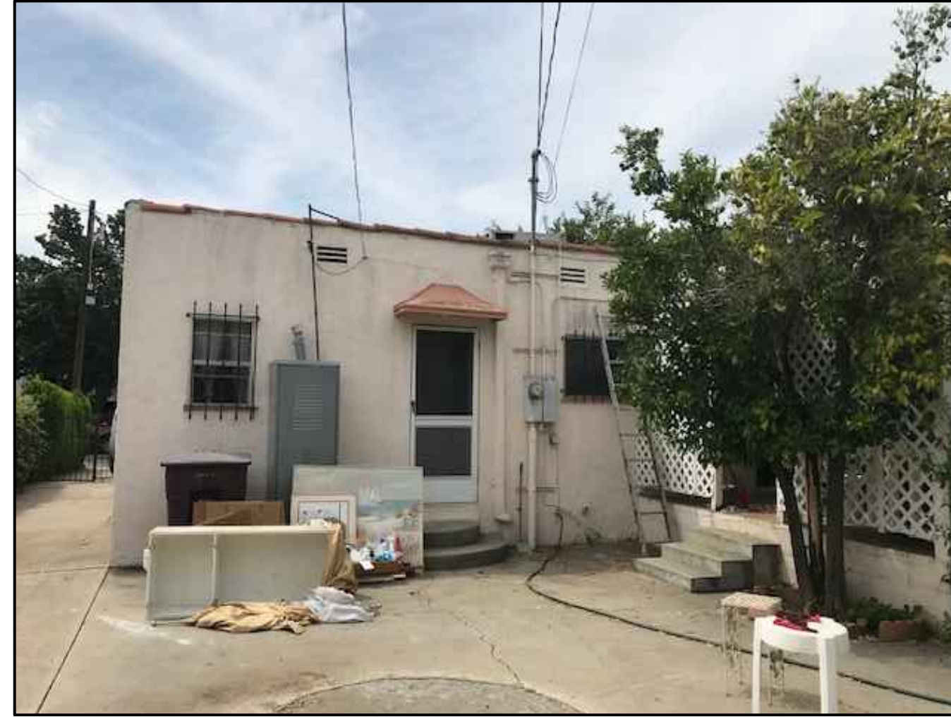
NORTH ELEVATION (partial rear view)
