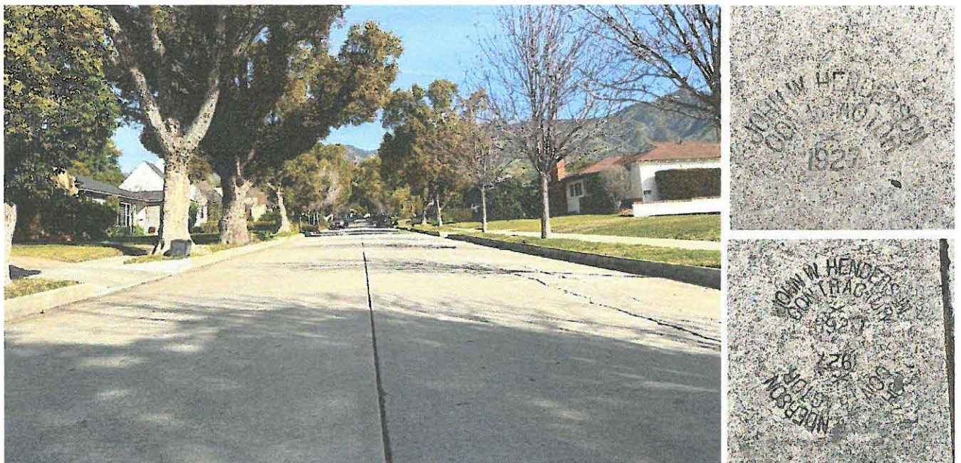
Exhibit 11. Idlewood Road with Original Macadam Surface and Street Stamp showing 1927 Construction Date
