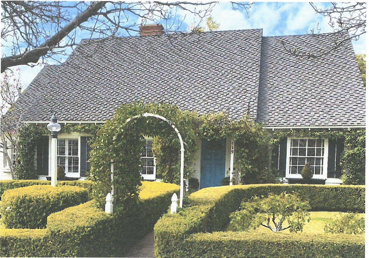
This 1940s home at 1419 Idlewood Road features the steeply pitched roof, clapboard siding, central chimney, and shutter-clad windows in a more or less rectangular shape of the Cape Cod revival style.
