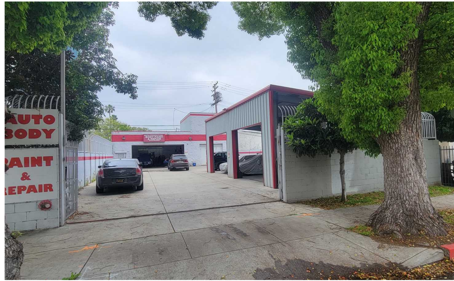
556 West Elk - note metal building
