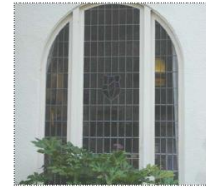
Above: This arched window has leaded glass. This opening is one of the most character defining on this house.
