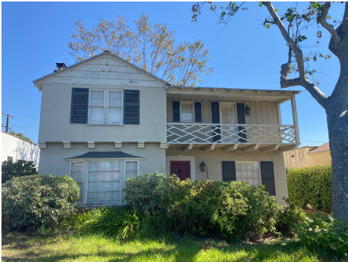
1334 Cleveland Road Monterey Revival
