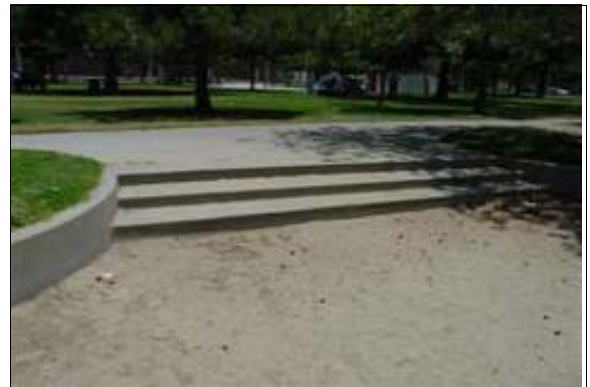
Exterior Stairs to the Play Area
