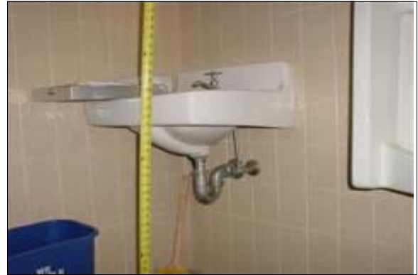
Unisex Restroom at the Maintenance Building
