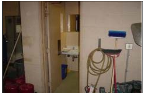
Unisex Restroom at the Maintenance Building
