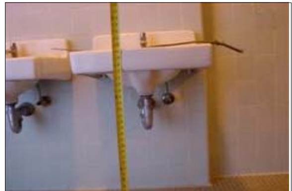
Women's Restroom at the Tennis Courts
