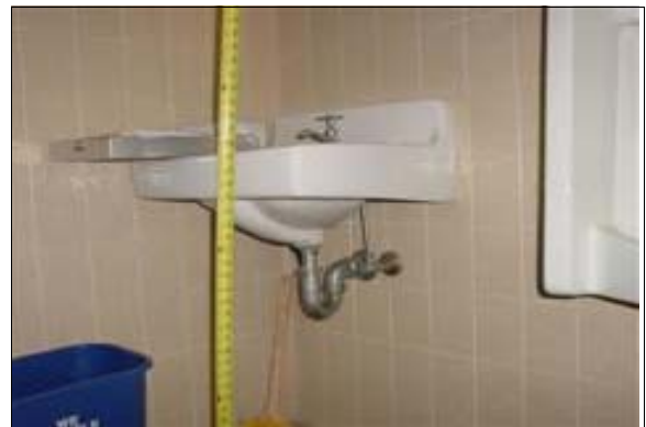
Unisex Restroom at the Maintenance Building
