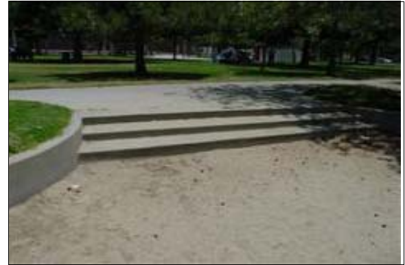
Exterior Stairs to the Play Area
