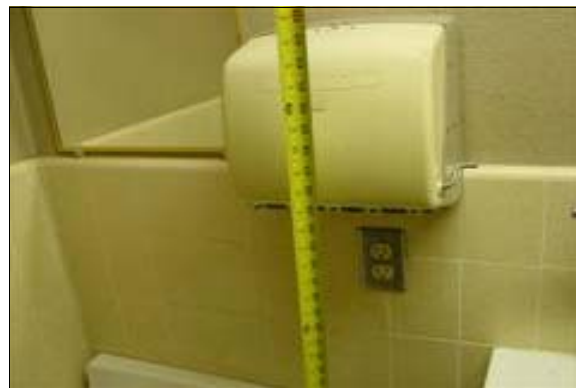
Unisex Restroom at the Maintenance Building
