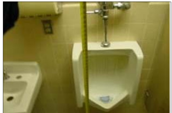
Unisex Restroom at the Maintenance Building
