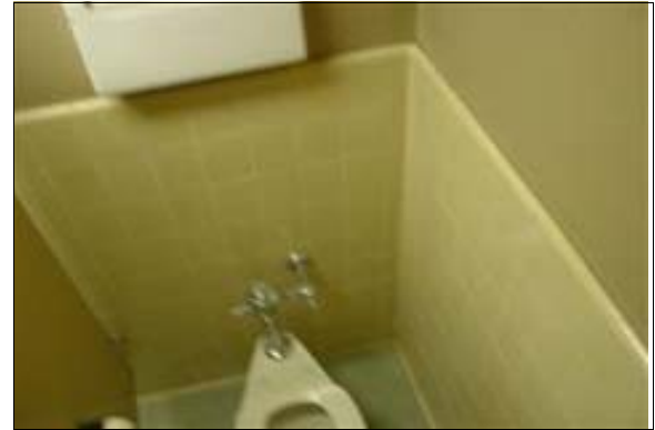
Unisex Restroom at the Maintenance Building
