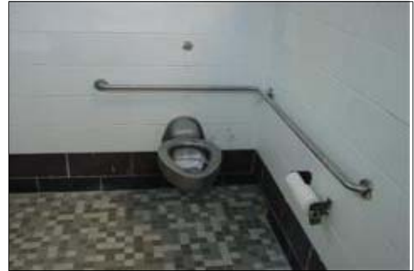
Men's Restroom Next to the Play Equipment
