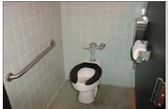
Women's Restroom at the Tennis Courts
