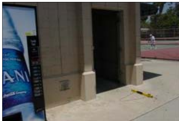
Women's Restroom at the Tennis Courts
