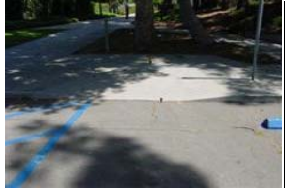
Curb Ramp at the Accessible Parking Space
