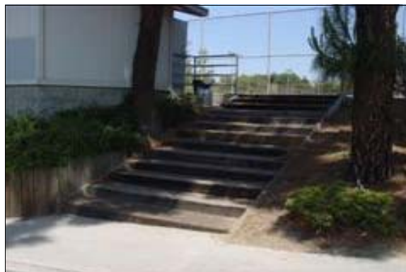
Exterior Stairs to the Tennis Courts
