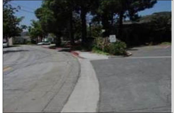
Curb Ramp off of Glorietta (Left)
