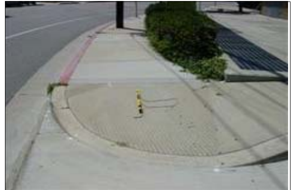
Curb Ramp off of Verdugo (Center Right)
