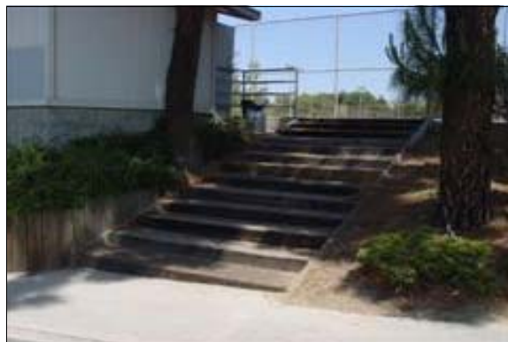
Exterior Stairs to the Tennis Courts
