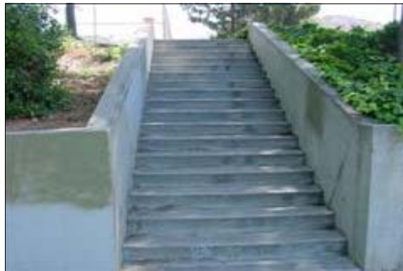
Exterior Stairs to the Tennis Courts
