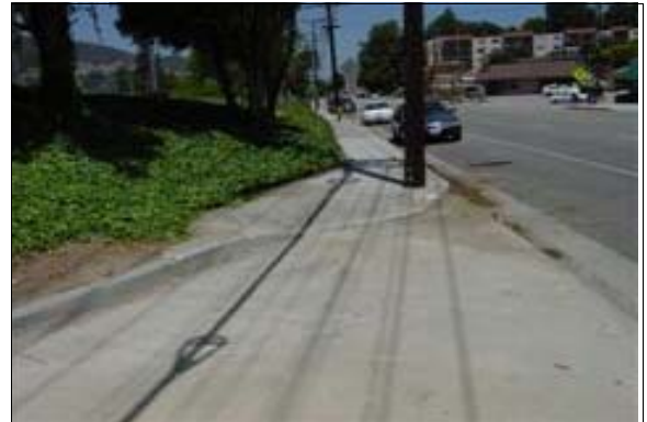
Curb Ramp off of Verdugo (Right)
