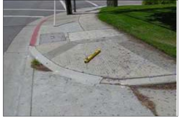
Curb Ramp off of Verdugo (Left)
