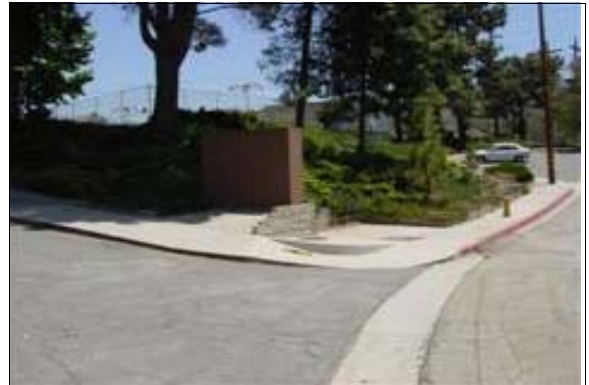
Curb Ramp off of Glorietta (Right)
