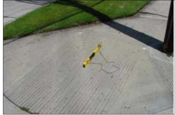
Curb Ramp off of Verdugo (Center Left)
