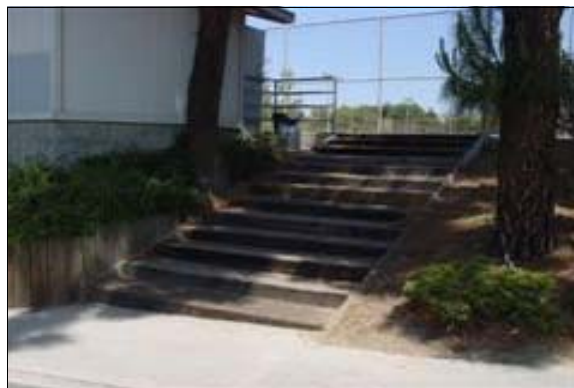
Exterior Stairs to the Tennis Courts
