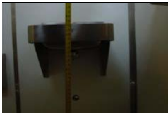
Unisex Restroom Next to the Community Center
