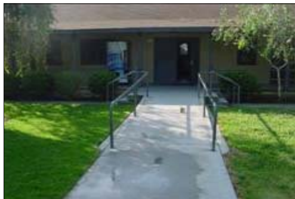
Exterior Ramp to the Community Center
