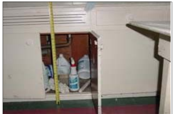
Sink in the Community Center
