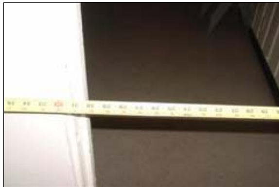
Interior Door in the Community Center
