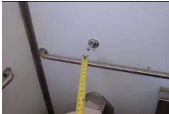
Unisex Restroom Next to the Community Center
