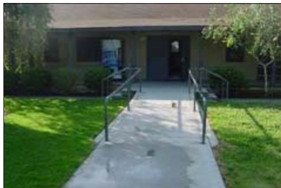
Exterior Ramp to the Community Center
