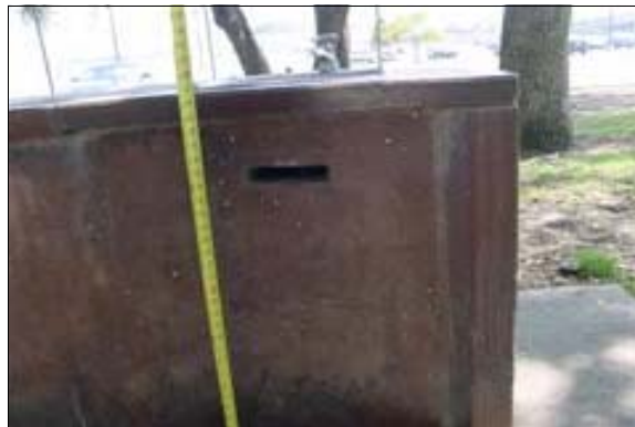
Sinks at the Covered Outdoor Dining Area
