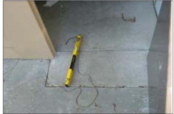
Unisex Restroom Next to the Community Center
