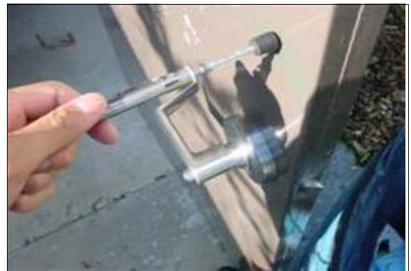
Unisex Restroom Next to the Community Center
