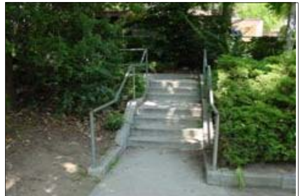
Exterior Stairs to the Lower Outdoor Dining Area (North)
