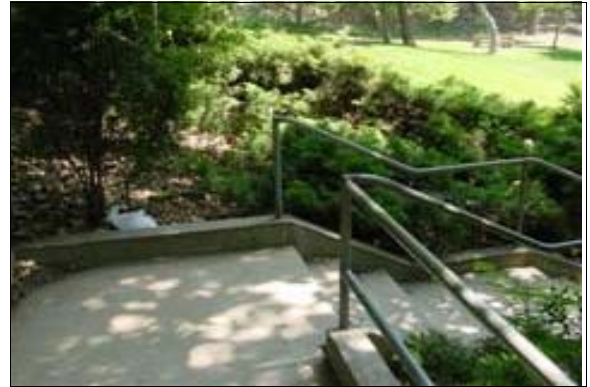
Exterior Stairs to the Lower Outdoor Dining Area (North)
