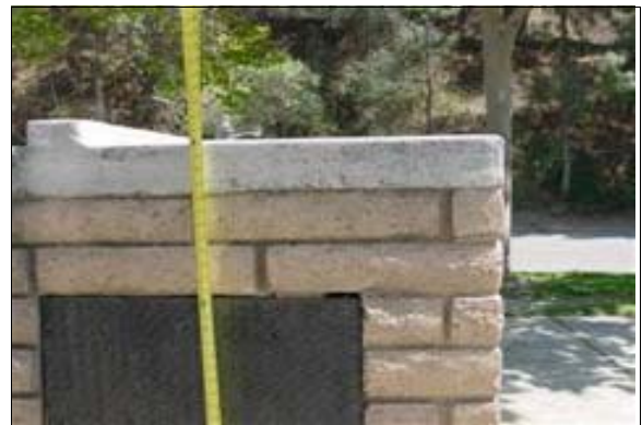
Sink at the Outdoor Dining Area
