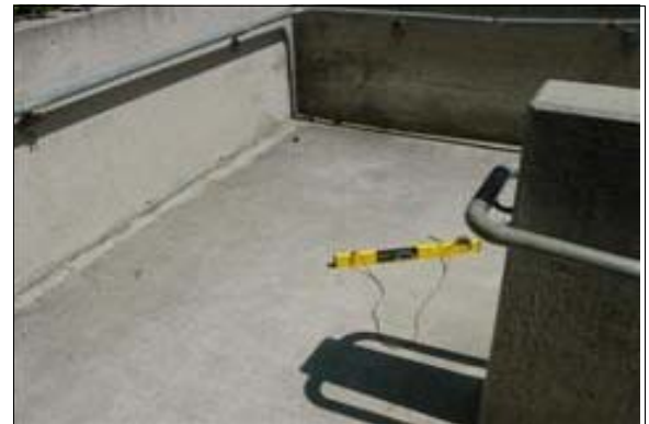
Exterior Ramp Next to the Restrooms
