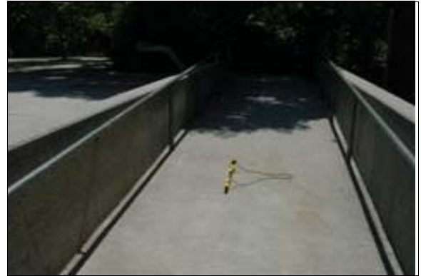
Exterior Ramp Next to the Restrooms
