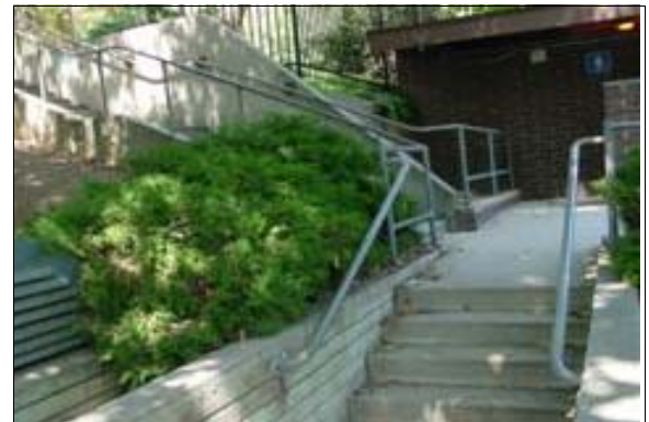
Exterior Stairs to the Play Equipment (Left)
