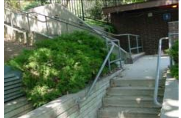
Exterior Stairs to the Play Equipment (Left)
