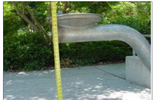
Drinking Fountain Next to the Restrooms
