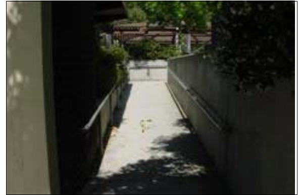
Exterior Ramp Next to the Restrooms
