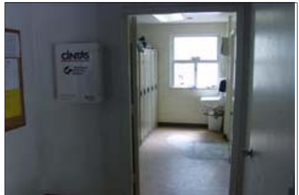
Unisex Restroom at the Maintenance Building
