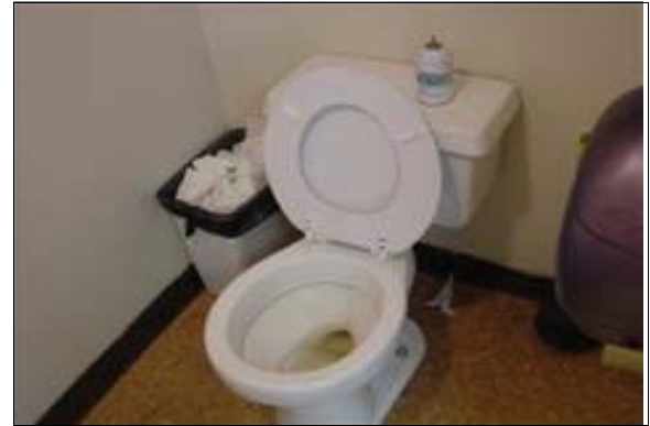
Unisex Restroom at the Maintenance Building
