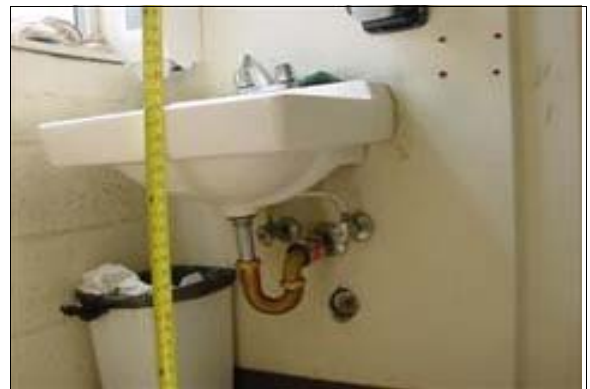
Unisex Restroom at the Maintenance Building
