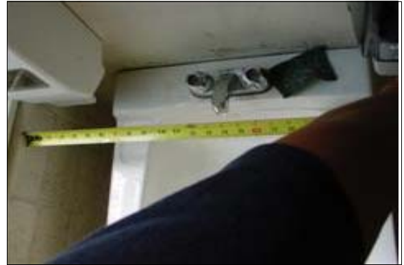
Unisex Restroom at the Maintenance Building
