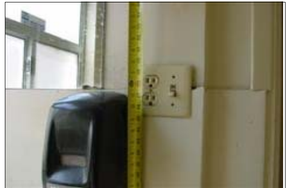
Unisex Restroom at the Maintenance Building
