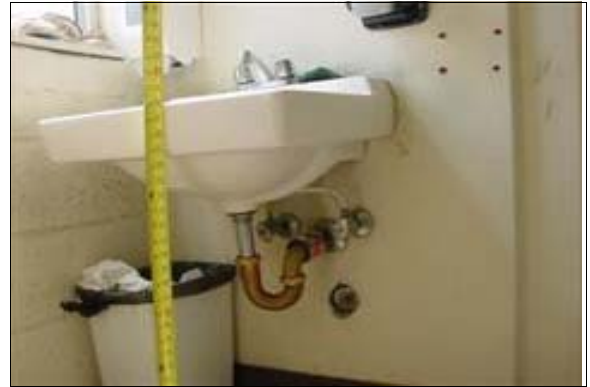
Unisex Restroom at the Maintenance Building
