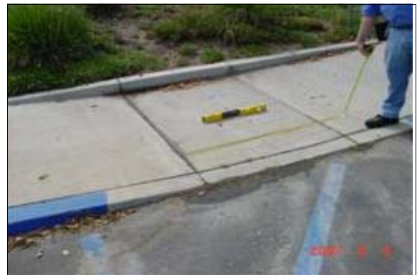
Curb Ramp at the Accessible Parking Spaces Next to the Baseball Field (Left)
