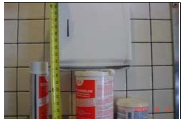
Unisex Restroom in the Maintenance Building
