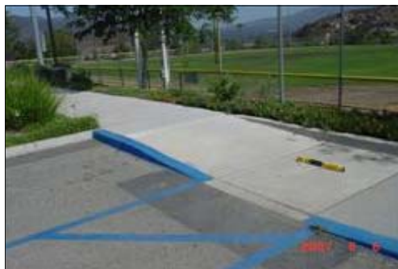
Curb Ramp at the Accessible Parking Spaces Outside of the Office (Left)
