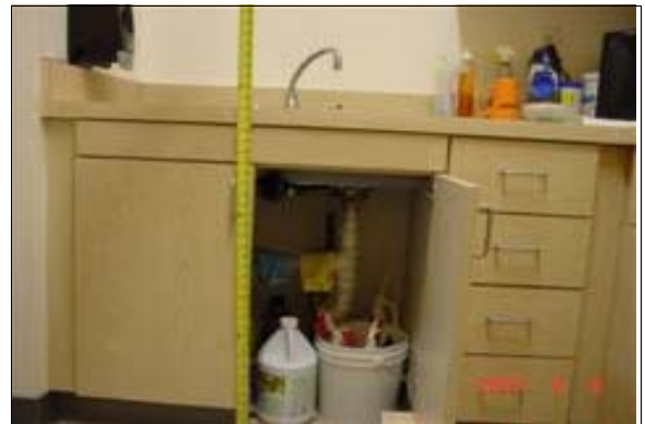
Sink in the Sports Complex Operations Office
