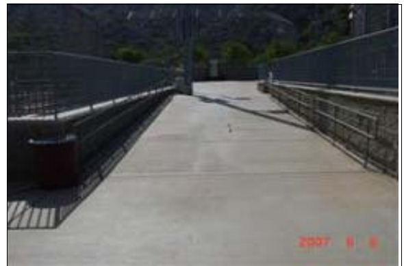
Exterior Ramp Between the Sports Fields
