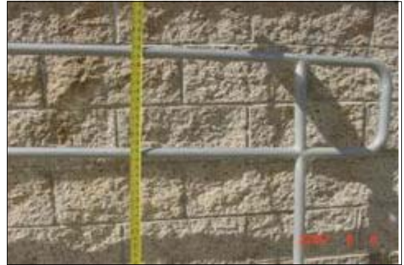
Exterior Ramp Between the Sports Fields
