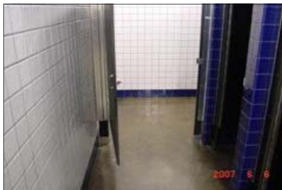
Women's Restroom at the Sports Complex Operations Office
