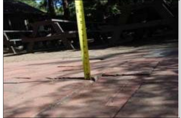
Path of Travel at the Outdoor Dining Area
