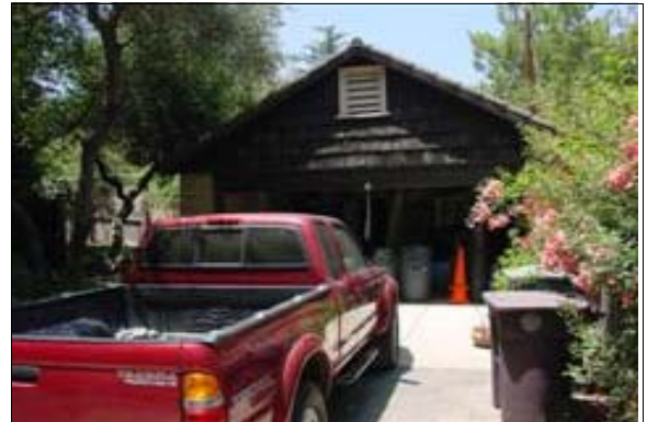
Path of Travel to the Maintenance Garage
