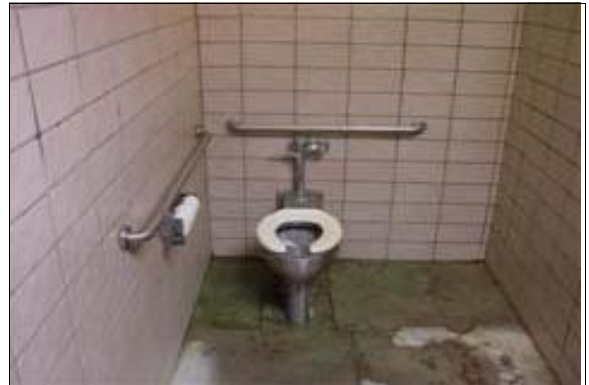
Men's South Restroom
