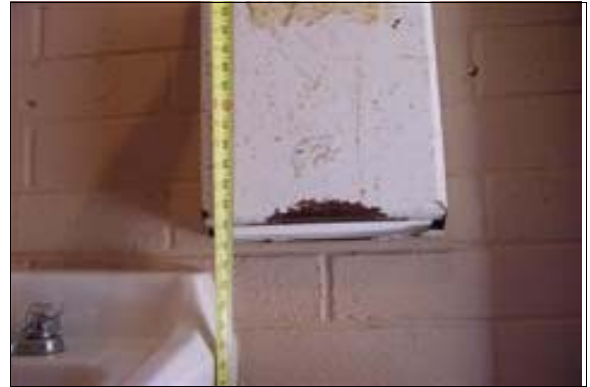
Unisex Restroom at the Maintenance Building
