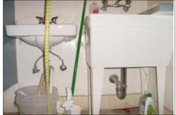
Men's Restroom in the High School Locker Room at Stengel Field
