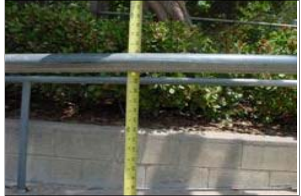
Exterior Ramp to Stengel Field
