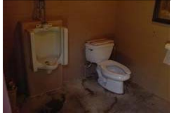
Unisex Restroom at the Maintenance Building
