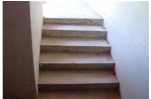
Exterior Stairs to the Locker Rooms at Stengel Field
