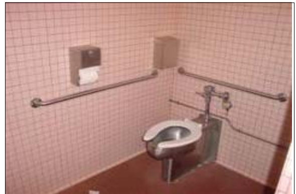
Women's Restroom at Stengel Field
