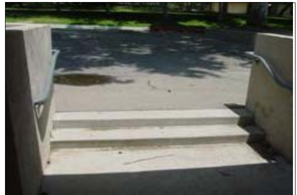
Exterior Stairs to the Restrooms at Stengel Field
