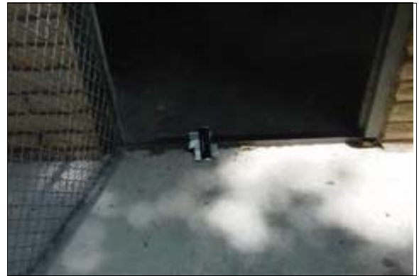
Food Service Building
