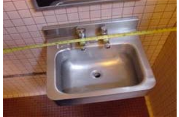
Women's Restroom at Stengel Field
