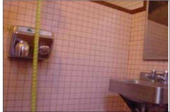
Women's Restroom at Stengel Field
