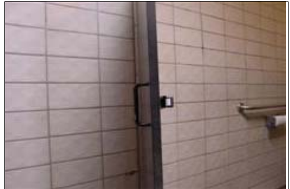
Men's South Restroom
