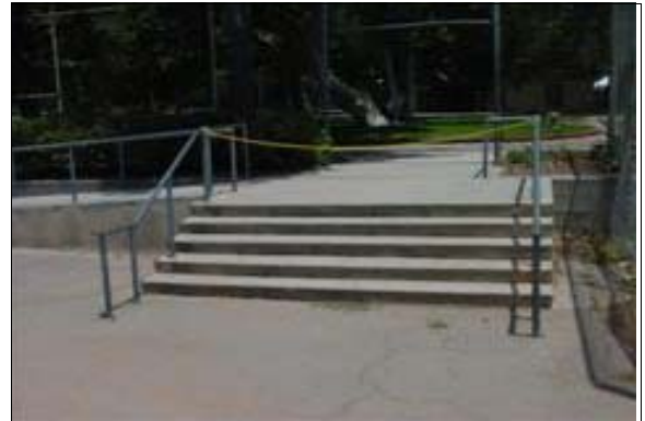
Exterior Stairs to Stengel Field
