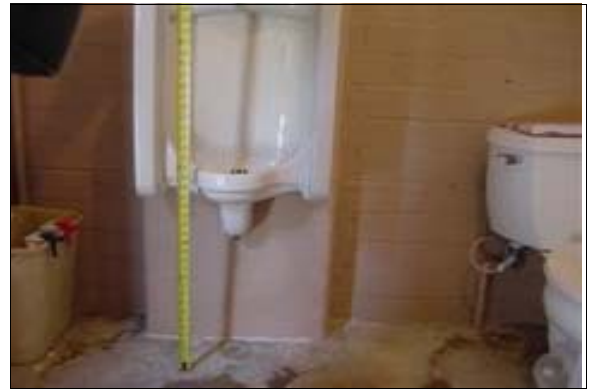
Unisex Restroom at the Maintenance Building
