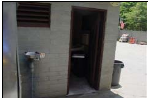
Unisex Restroom at the Maintenance Building
