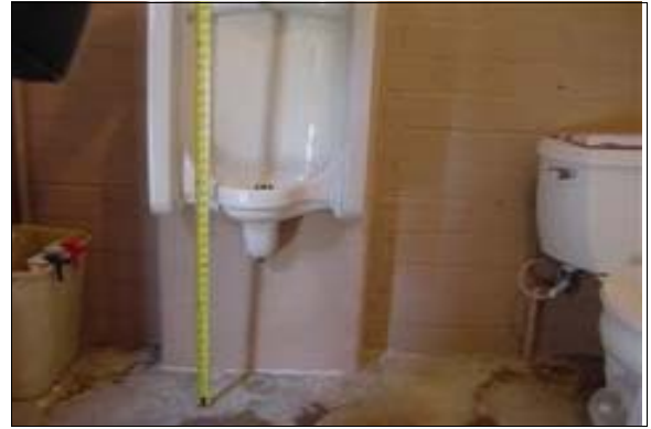
Unisex Restroom at the Maintenance Building
