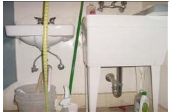
Men's Restroom in the High School Locker Room at Stengel Field
