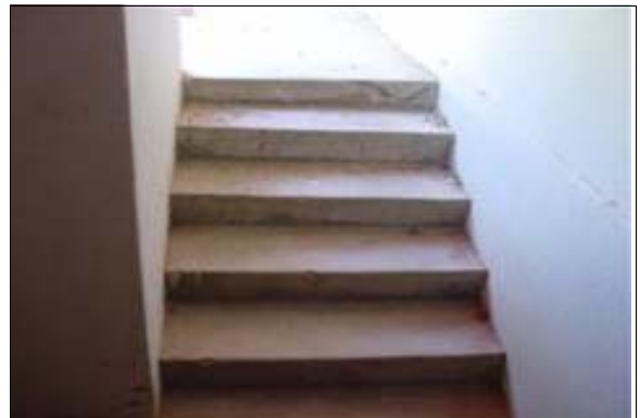
Exterior Stairs to the Locker Rooms at Stengel Field
