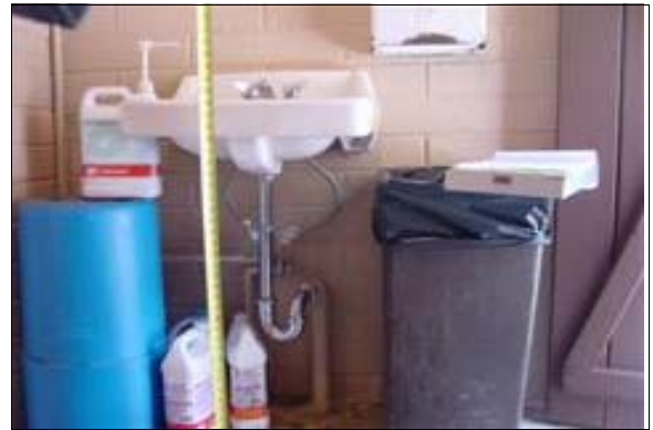
Unisex Restroom at the Maintenance Building
