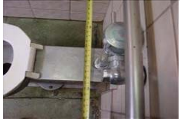
Men's South Restroom
