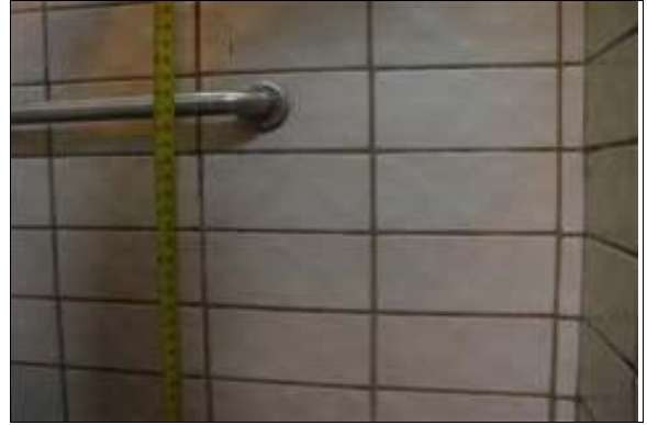
Men's South Restroom
