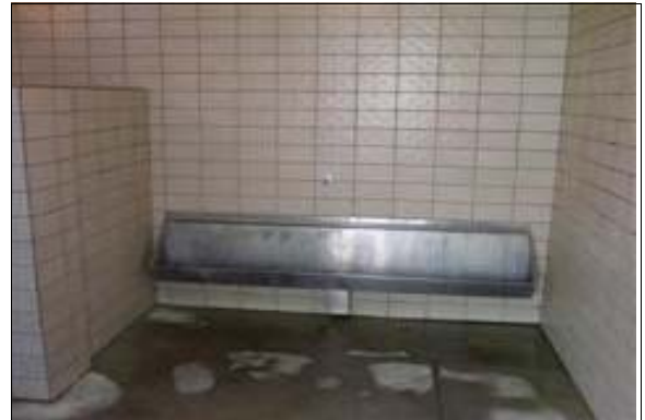
Men's South Restroom
