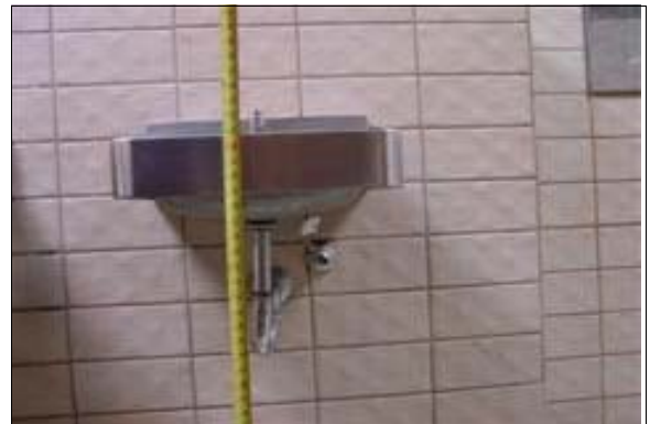
Men's South Restroom
