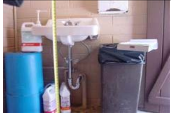
Unisex Restroom at the Maintenance Building
