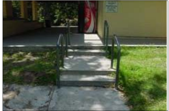
Exterior Stairs to the North Restrooms
