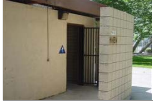
Men's South Restroom
