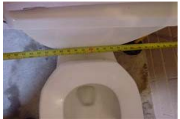
Unisex Restroom at the Maintenance Building
