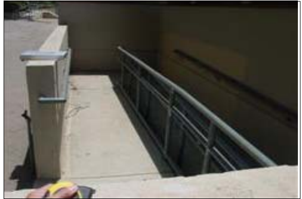
Path of Travel to the Restrooms at Stengel Field
