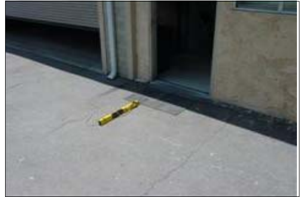
Path of Travel to the Maintenance Building
