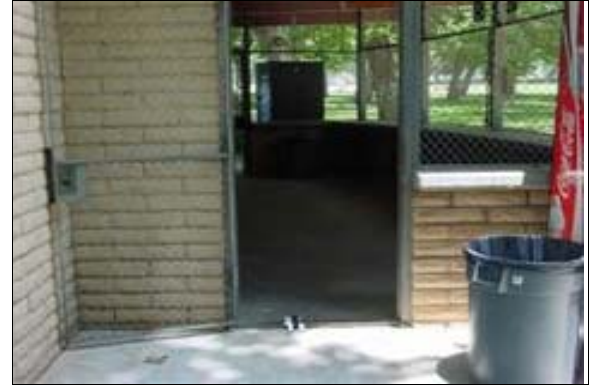
Food Service Building
