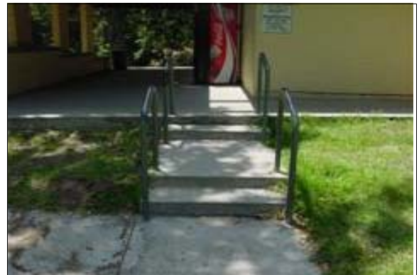
Exterior Stairs to the North Restrooms
