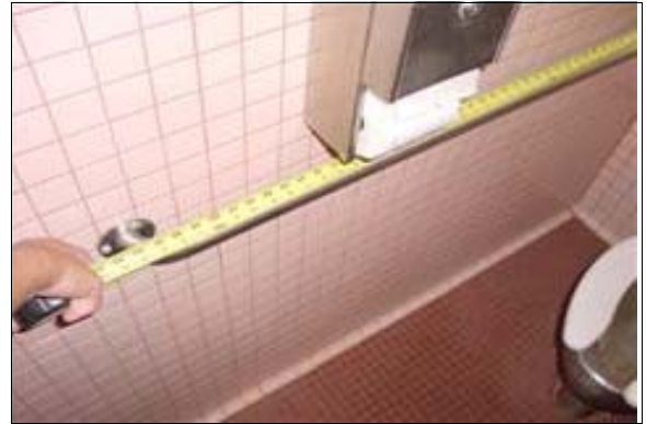
Women's Restroom at Stengel Field
