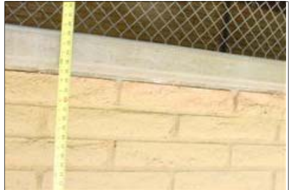
Food Service Building
