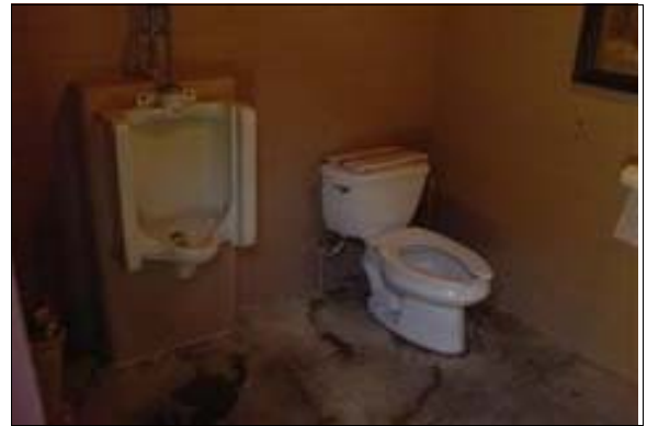
Unisex Restroom at the Maintenance Building
