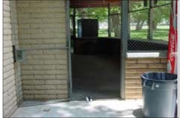
Food Service Building
