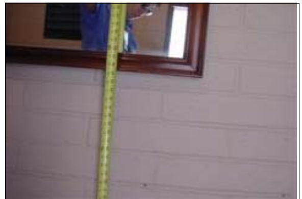
Unisex Restroom at the Maintenance Building
