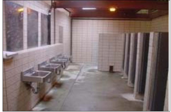
Men's South Restroom
