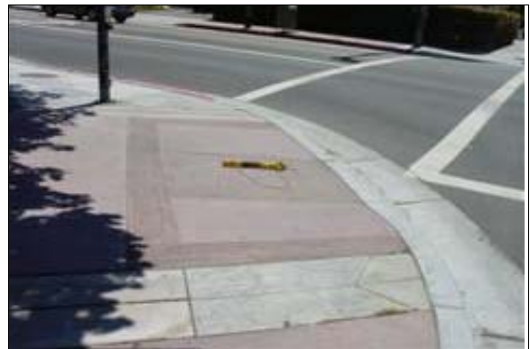
Curb Ramp at the Corner of Wilson and Adams
