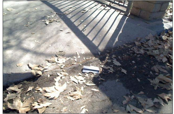
Curb Ramp at the Accessible Parking Access Aisle
