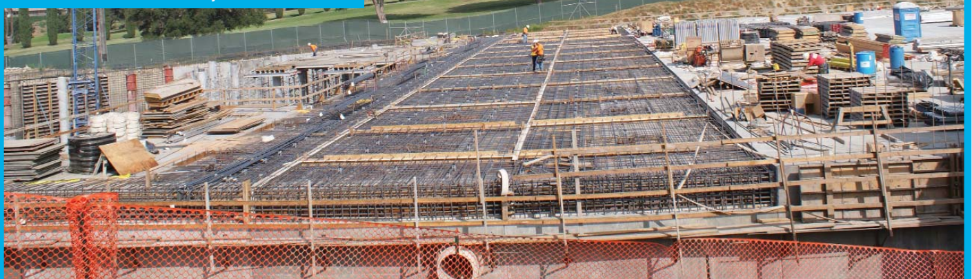
Refurbishment of the Chevy Chase Reservoir
